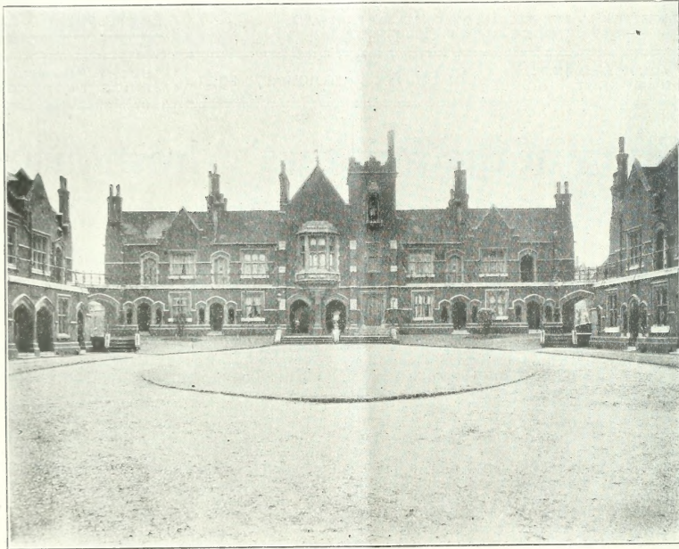
THE PRINTERS' ALMSHOUSES AT WOOD GREEN.
