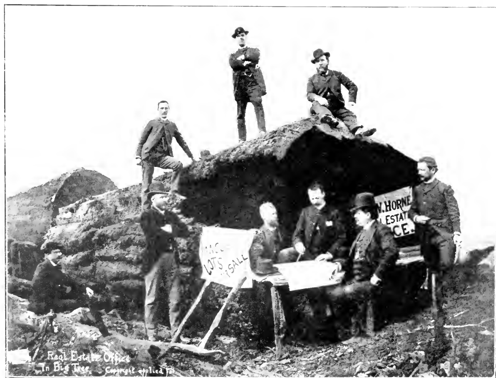
J. W. HORNE'S REAL ESTATE OFFICE, AFTER THE VANCOUVER FIRE
