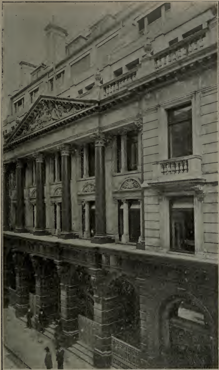
THE NEW BALTIC—EXTERIOR VIEW FROM ST. MARY AXE
