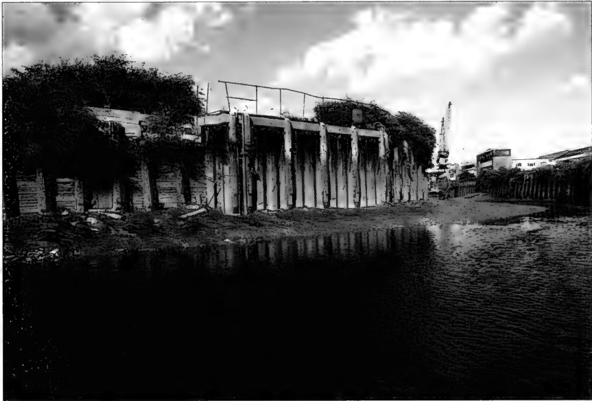
Fig. 2. General view of the central reach of Deptford Creek, looking north. The tide is about half out, and the silt mudbanks are beginning to be exposed. At low tide, the water is confined to a small flowing channel in the centre of the creek, about 3 metres wide and 30 cm deep. Buddleia grows out from the tops of the wharfs, there is some sprouting vegetation from the old timber frontages (left and far distance), but virtually none from the sterile sheet metal piling (centre). Photo N. Bertrand.
