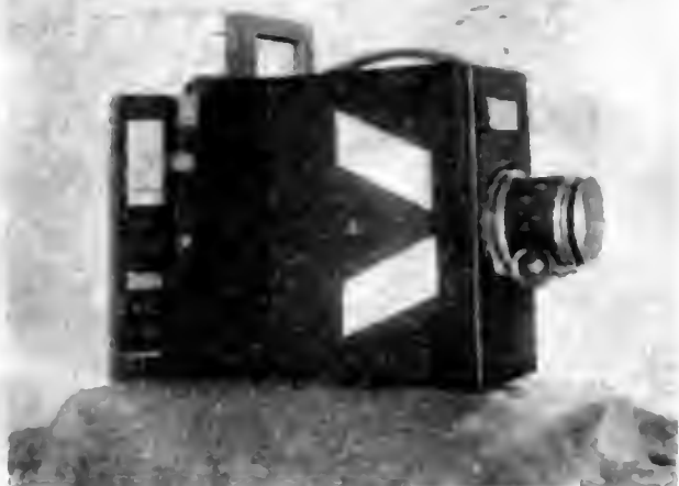
Fig. 1.—Camera made according to Patent 12,181 of 1909. Position and shape of prisms are shown by pieces of paper attached to camera. Filter holders and dark-slide resting against back of camera.
