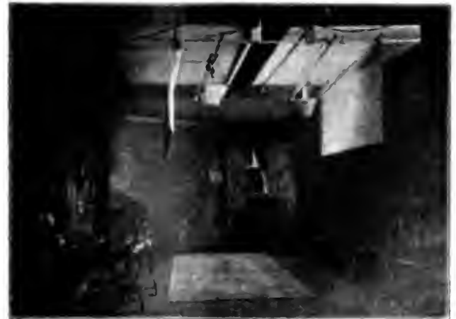
Fig. 1. Photograph of Mr. T. C. Turner's studio, showing adjustable reflectors mounted on rollers placed on each side of the half-watt installation and movable transversely.
