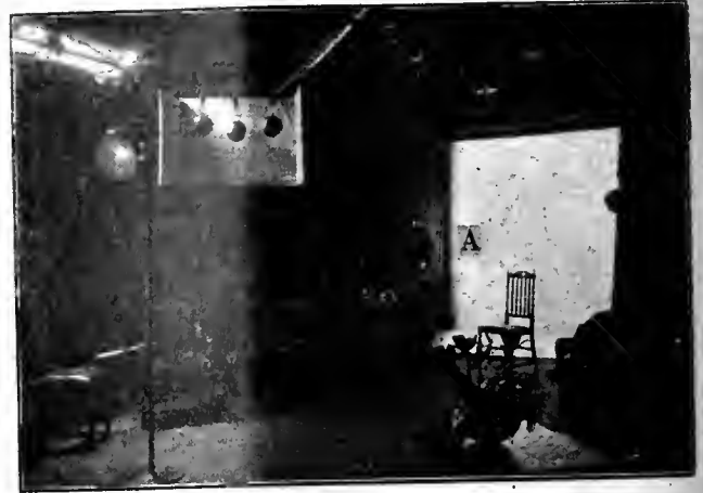
Fig. 4.—Photograph showing system of main lighting with three 1,500-watt lamps. The white background is shown as used for sketch portraits, being lighted by a G.E.C. flood light lamp shown at A.
