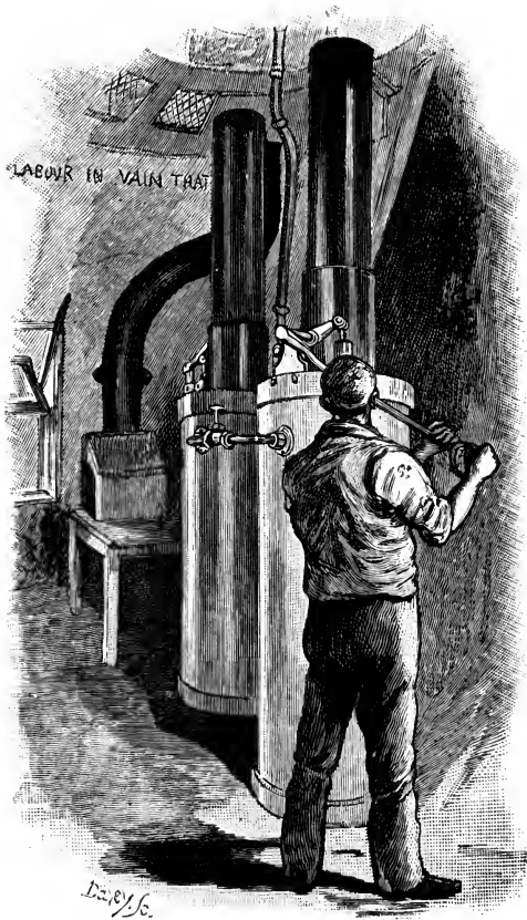
PUMPS FOR FORCING THE OIL UP TO THE LAMPS AT THE EDDYSTONE LIGHTHOUSE.
