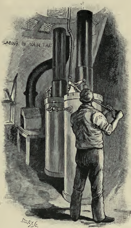
PUMPS FOR FORCING THE OIL UP TO THE LAMPS AT THE EDDYSTONE LIGHTHOUSE.
