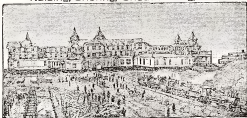
Moving Brighton Beach Hotel in 1888. Length 460 feet, Depth 210 feet, Weight 5,000 tons. B. C. MILLER Telephone 1514 Prospect ALBERT E. MILLER
