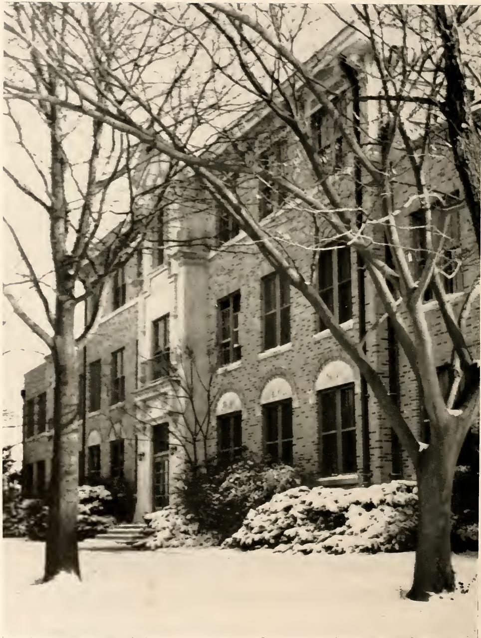
SNOW SCENE, BROOM ADMINISTRATION BUILDING
