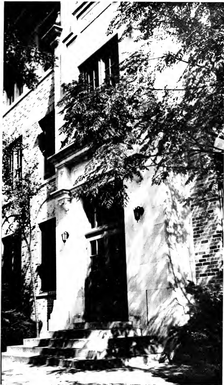
BROOM MEMORIAL ADMINISTRATION BUILDING
