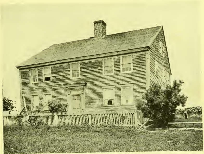
House Built by Elder Simeon Brown (72) Near the Second Baptist Church, North Stonington, Conn. This house appears the same as it did in 1836, when Josiah (279) and his wife lived here with his son, Josiah, Jr. (304). Afterwards owned by Ira (390). Now, August, 1907, it is owned by Angeline (Brown) Vincent (392)
