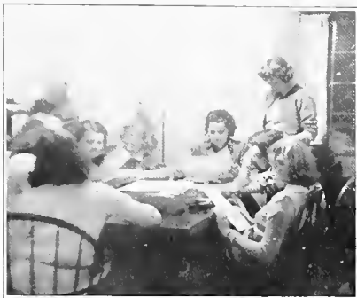
THE NEW BOARD "... set about renovating the Notes "
