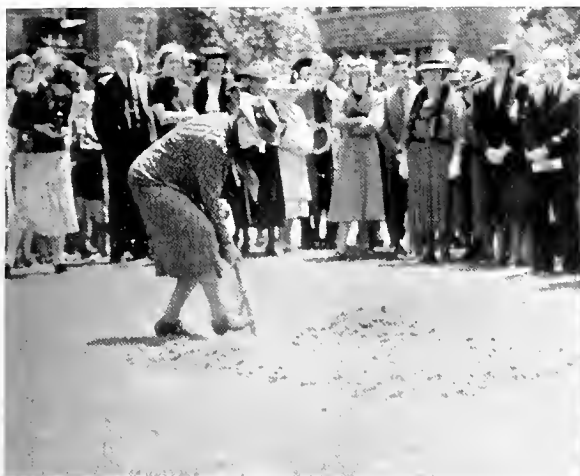
Ground Breaking: May, 1938
