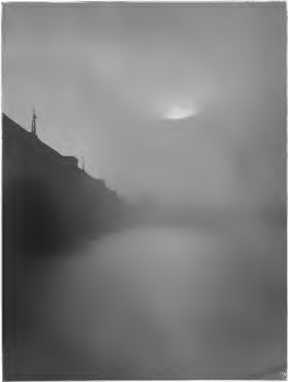
Waterloo Bridge - London
