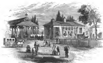
STATION AT CASTEL, OPPOSITE MAINZ, FRONT VIEW
