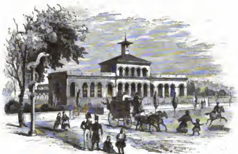
STATION AT WIESBADEN, VIEW FROM THE STREET.
