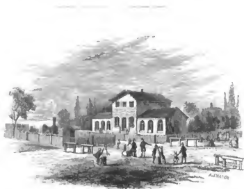
STATION AT HÖCHST, VIEW FROM THE RAILWAY.
