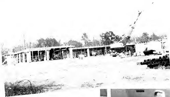
Construction begins on the new men's dormitory on South Campus.
