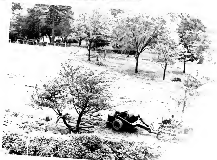
Bulldozer clears arboretum for construction of new classroom building.
