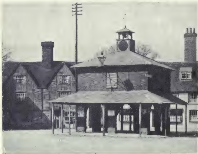
Market House, Princes Risborough
