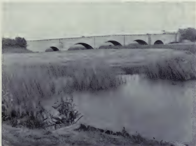
Bridge over the Ouse at Olney
