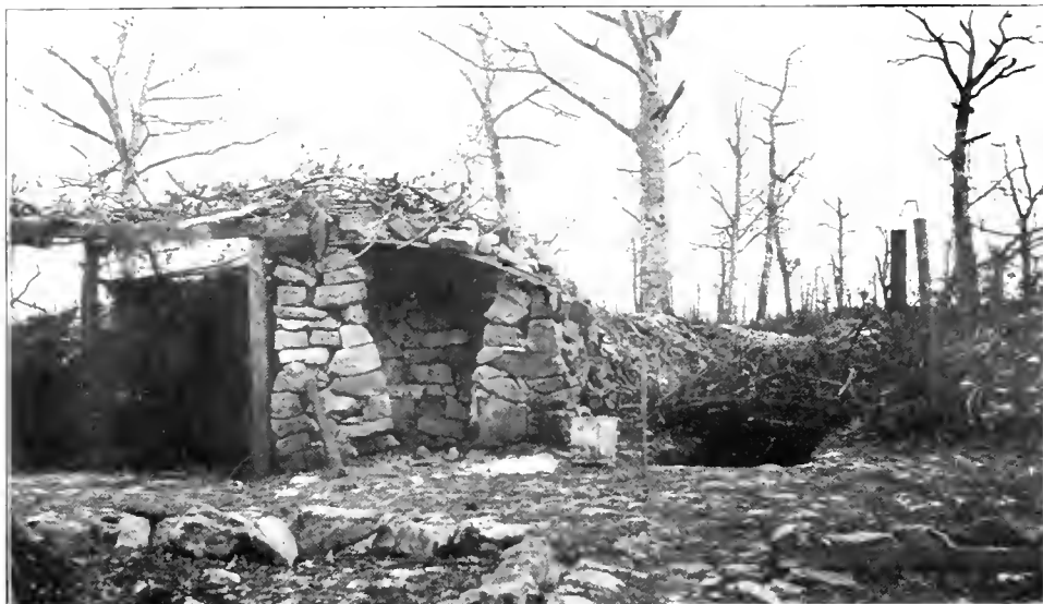
A typical German dug-out, occupied by the Yanks after its capture. The shelter at the left of the entrance protected the gas guard at night from flying shell fragments. Suspended from the post at the right is a short length of railroad rail used as a gas alarm. In the left hand corner can be seen a "dud," a shell that failed to explode.
