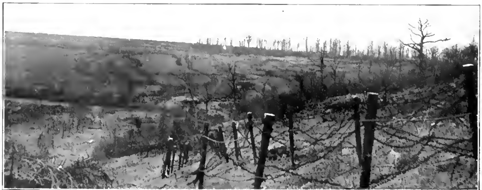
Barbed wire entanglements in the St. Mihiel Sector. Mostly of German construction, but later rebuilt and strengthened by the Yanks to hold off German counter-attacks. The irregular lines in the distance are successive waves of wire
