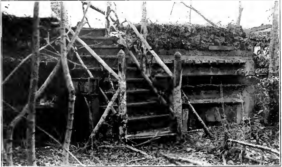
A German officers' dug-out—a stronghold built of successive layers of steel and concrete several feet in thickness
