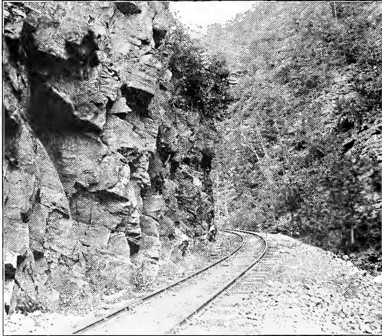
VIEWS ALONG THE NARROW GAUGE
