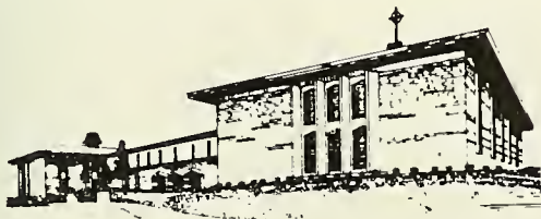
The B. D. Phillips Memorial Building
