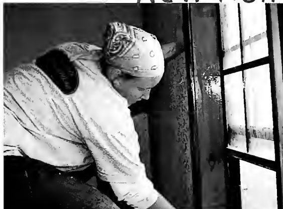
Sophomore Brandi Franklin puts the final coat of stain around a window of one of the new houses. This was Franklin's second trip to Mexico and could not wait to return and complete more projects.
