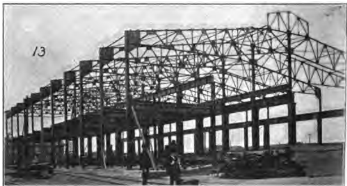
Half of Steel Framework of No. 7
