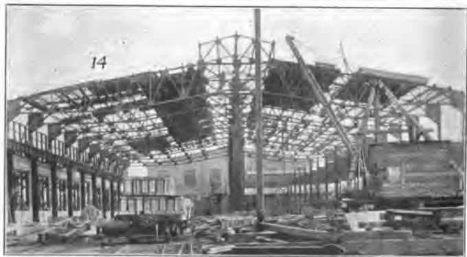
Part of Steel Framework of U. P. R. R. Boiler Shop
