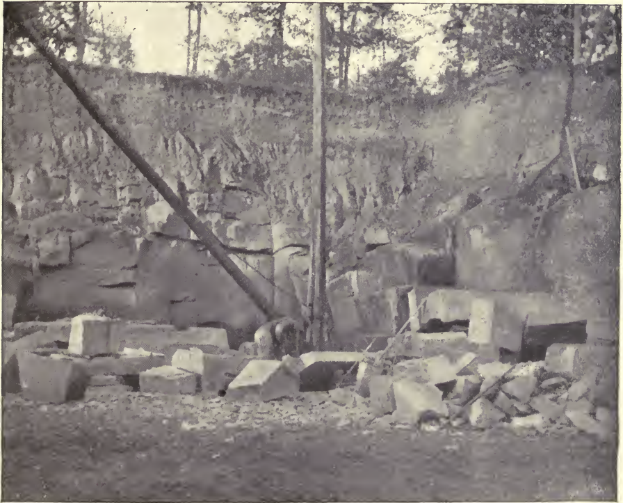
Fig. 6.—Mitchell's Quarry, Newtown, Pa., showing thickness of layers, system of jointing and amount of stripping.
