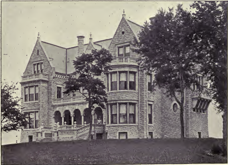
J. H. Sternberg's residence, Reading, Pa. Berks county pink sandstone. Showing Pennsylvania brownstones in public and private buildings.
