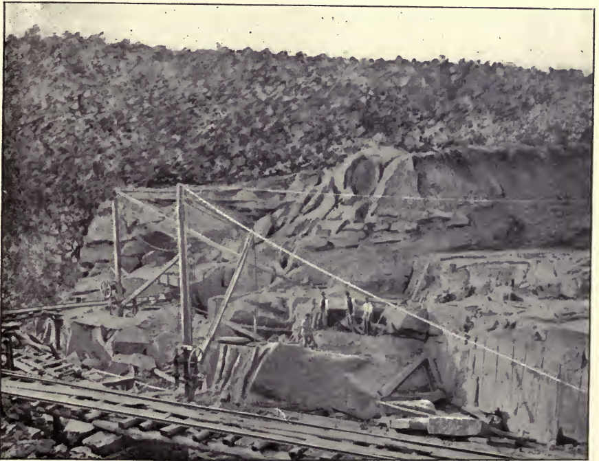
View in John Westley's quarry, Mohnsville, Pa. Showing structure of the stone and method of working.
