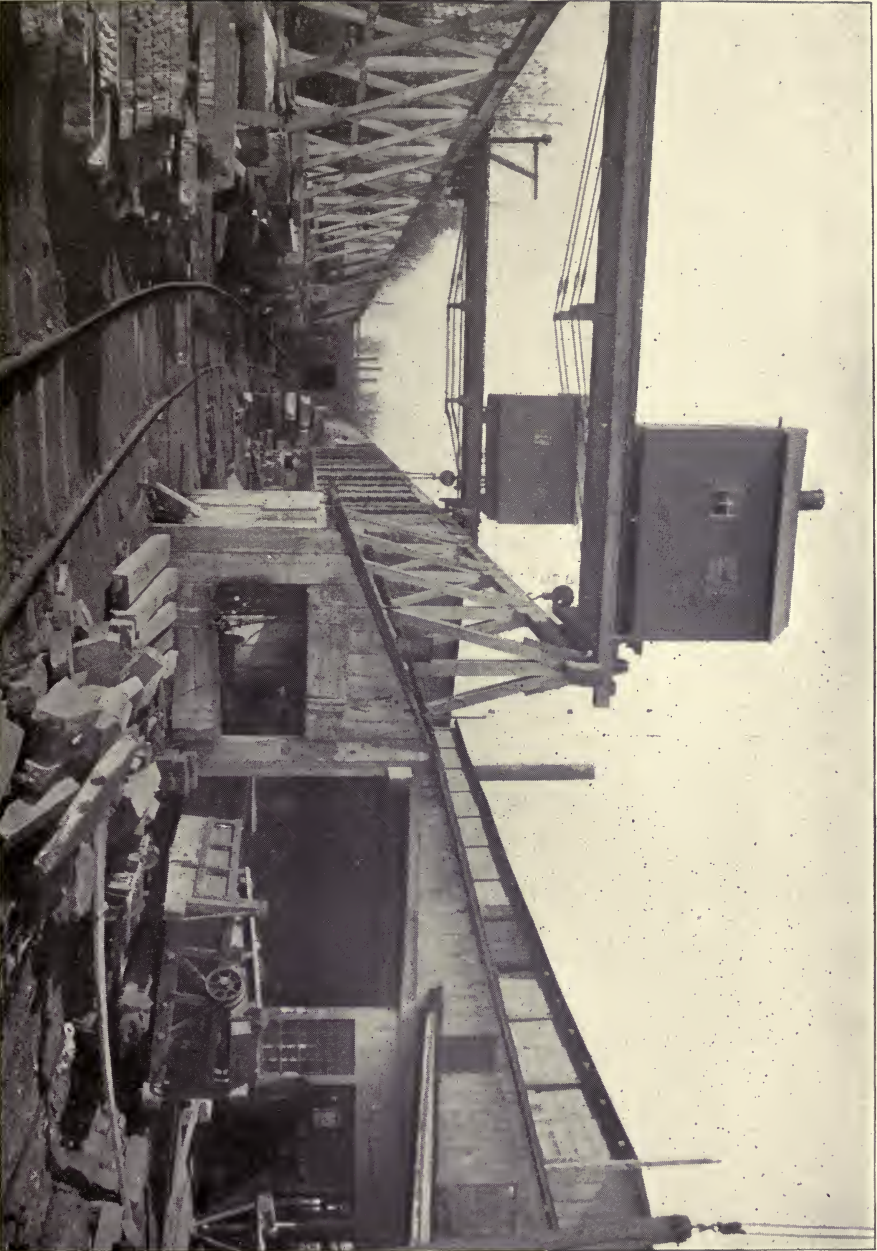
View of the stone sawmill and stream travellers for handling the stone at the Hummelstown Brownstone Company's Yard.
