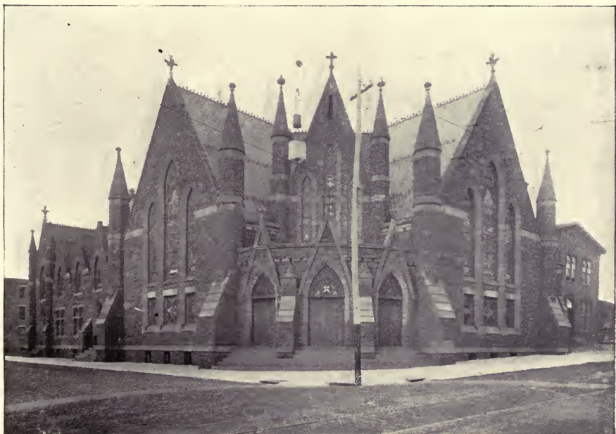
Westminster Presbyterian Church, Harrisburg, Pa. Showing the use of Hummelstown brownstone in public buildings.
