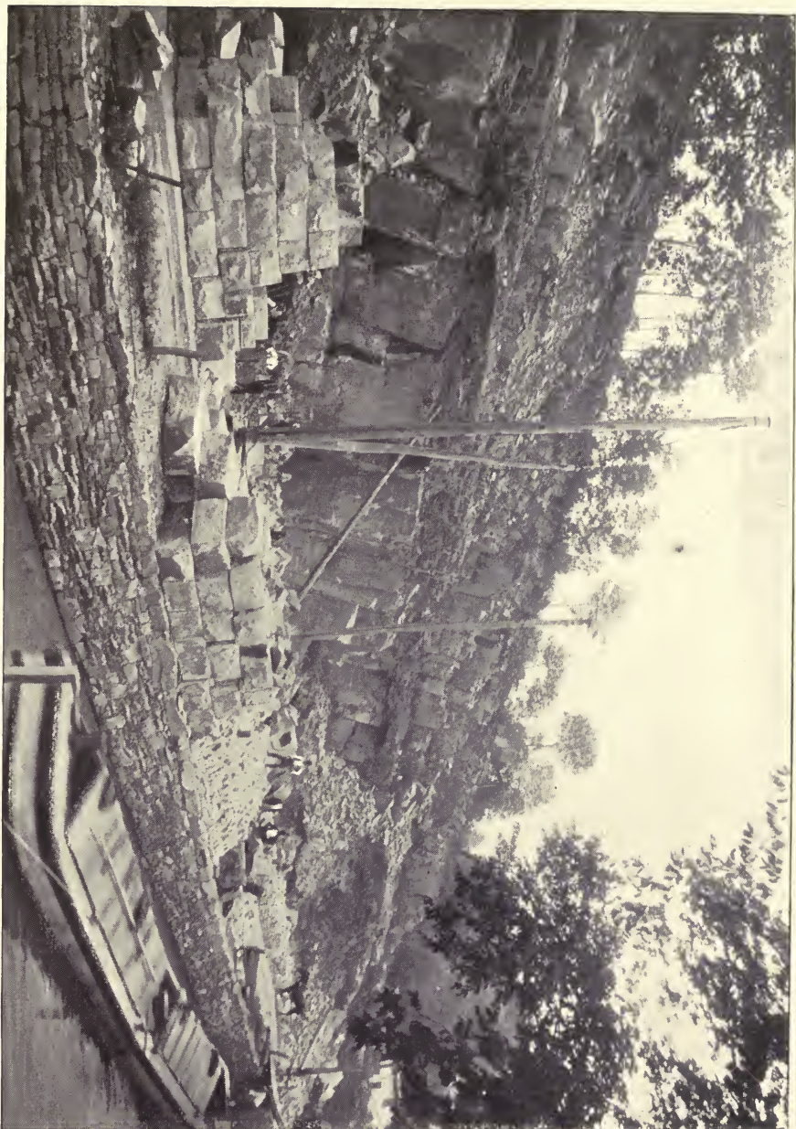
Paxson's Quarry, Jumberton, Pa., Showing structure of the stone and facilities for loading and shipping.
