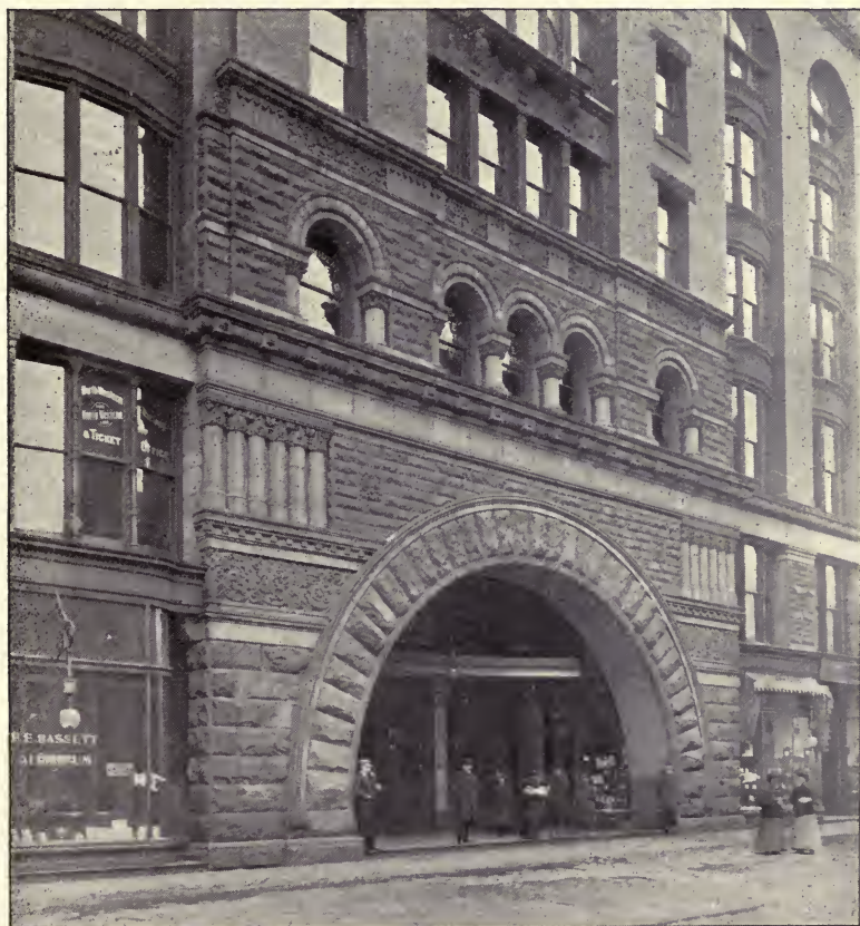
Arcade Building, Cleveland, O., and enlarged view of the entrance. Entrance, piers and trimmings of Hummelstown brownstone.
