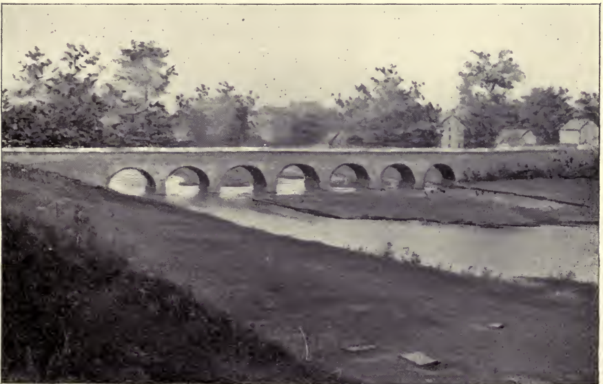
2. Bridge at Edison, Pa., built in 1800 of stone from the neighboring hills.
