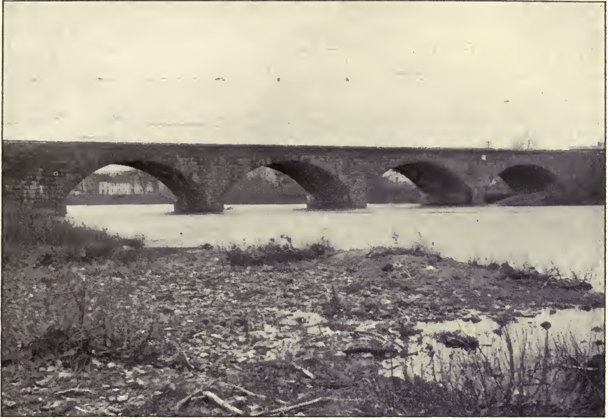
1. Pennsylvania Railroad bridge at Middletown, Pa., of Hummelstown brownstone.
