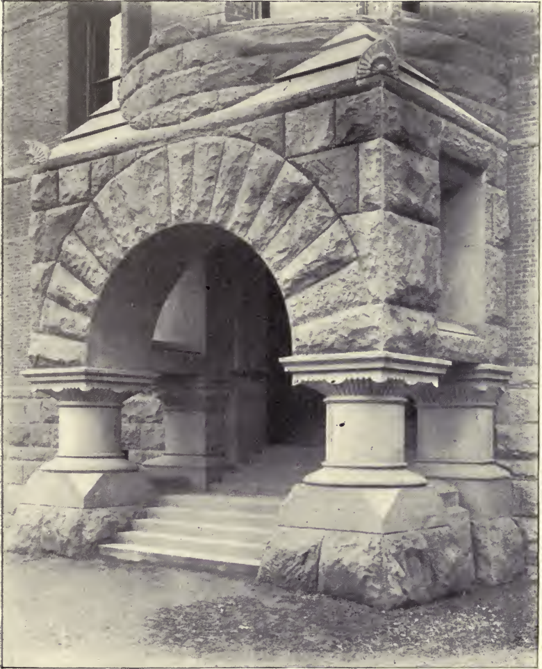
Entrance to Engineering Building, State College, Pa. Showing the use of Hummelstown brownstone in doorways.
