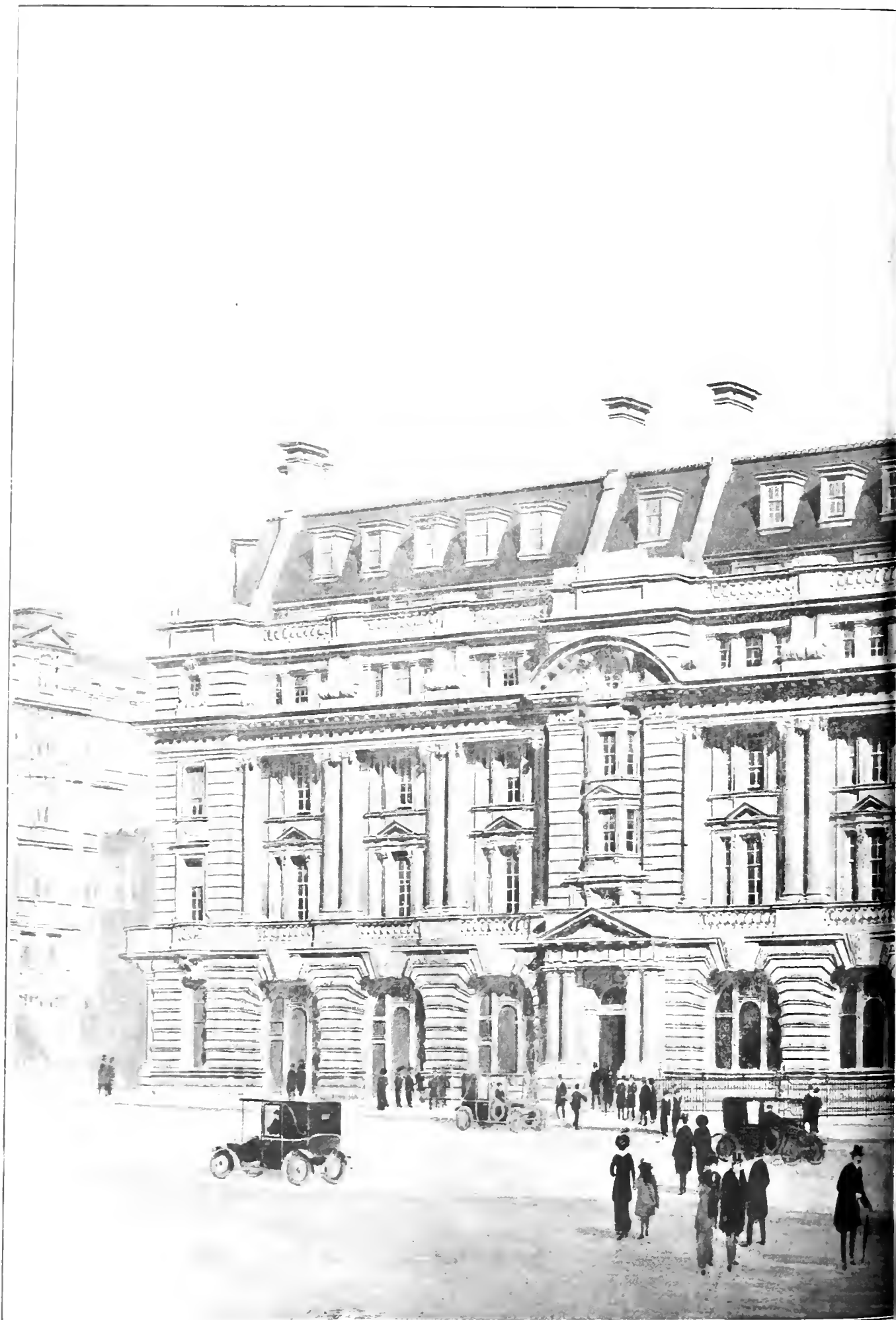
MESSRS. LLOYDS' NEW BANK, ST. JAMES'S STREET, S.W.—5575
