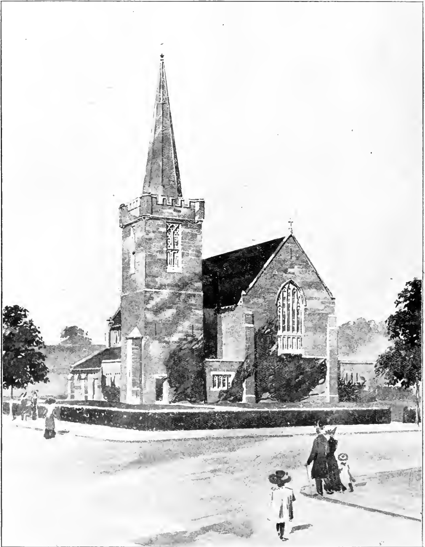
CHURCH OF ST. LUKE, THORNTON HEATH, SURREY. Mr. WILLIAM A. PITE, F.R.I.B.A., Architect.
