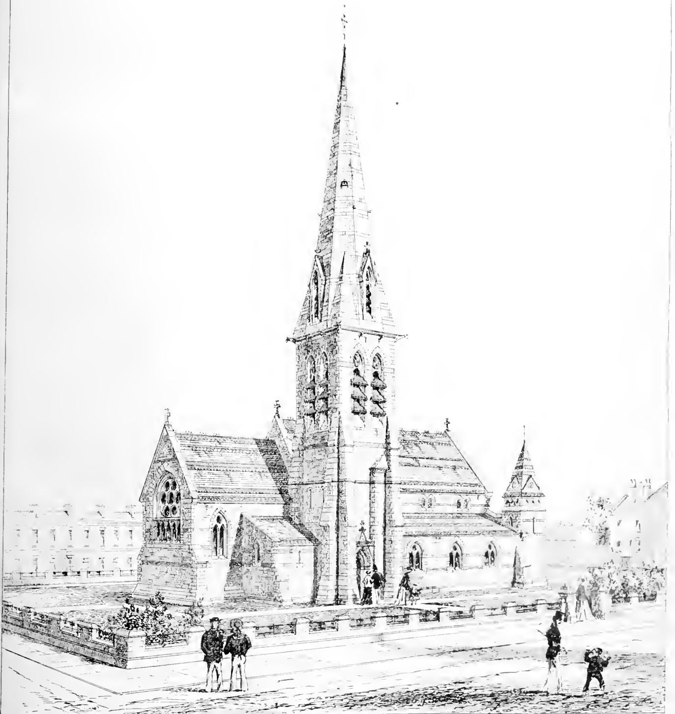
St. Luke's Church, Millwall. — M r E. L. BLACKBURNE, ARCHT.
