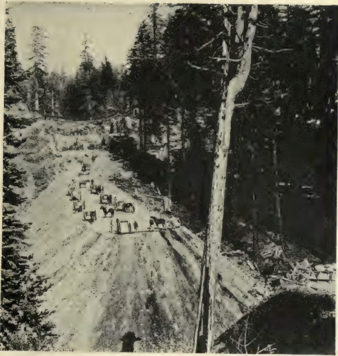
BUILDING THROUGH THE FOREST Central Pacific R. R., Sierra Nevada Mountains, 1864
