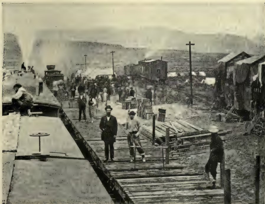
CENTRAL PACIFIC CONSTRUCTION CAMP, 1869 Chief Engineer Montague is the bearded man in center
