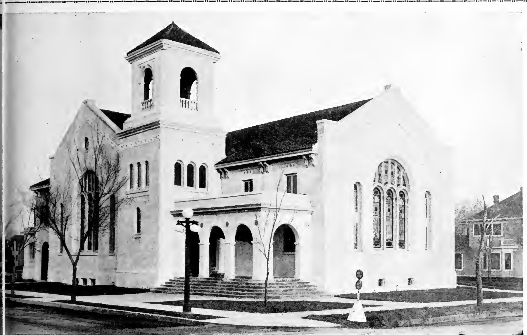
ROOFED WITH SIMONS LARGE SPANISH TILE.
