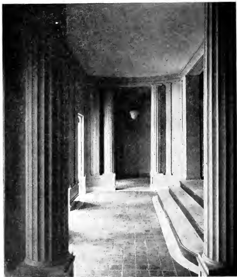
MAIN ENTRANCE VESTIBULE, MARIAN GRAMMAR SCHOOL, LOS ANGELES, CALIFORNIA.
