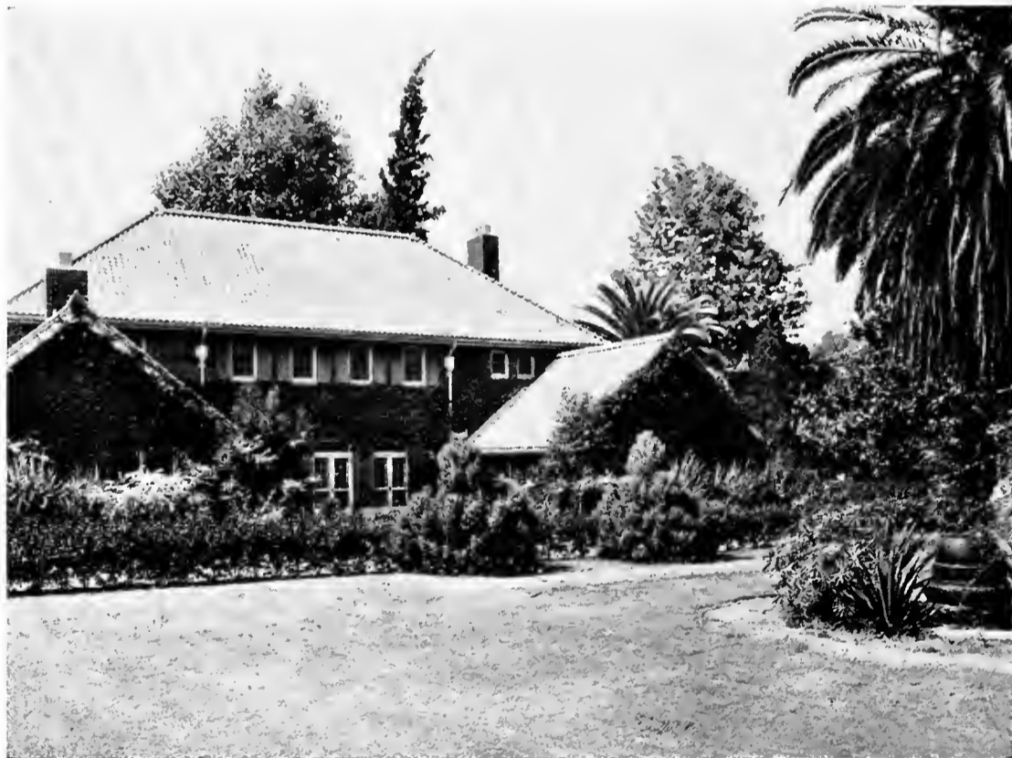
REAR OF BOYS COTTAGE No. 10
