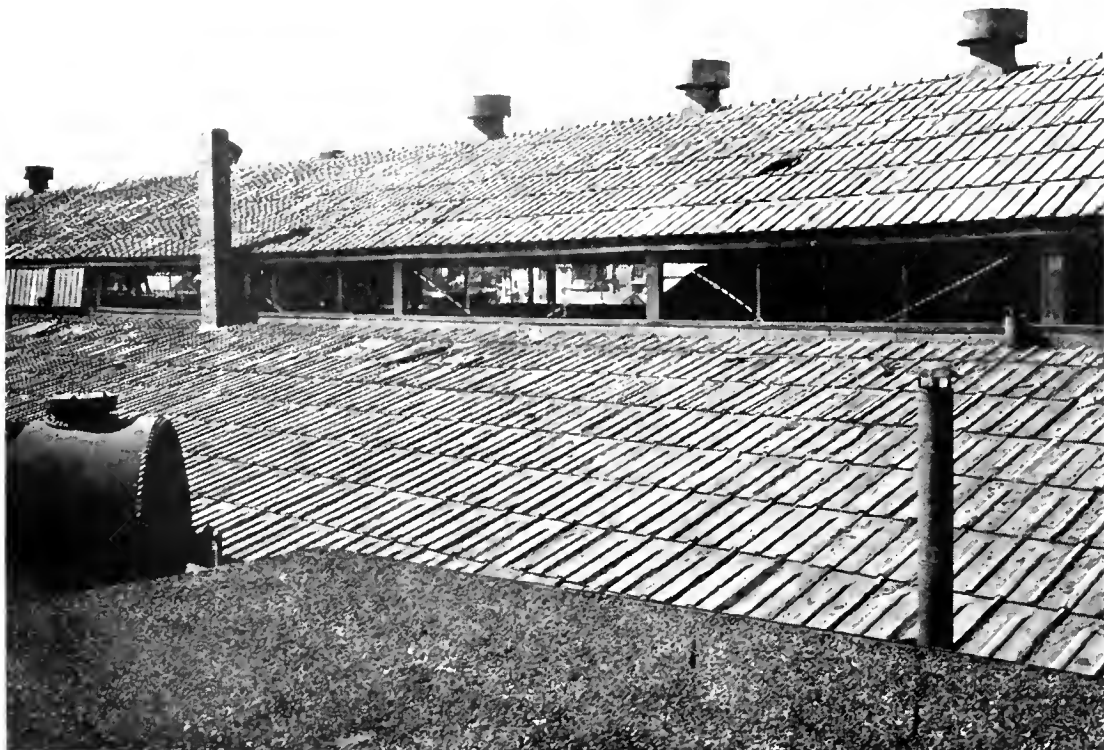
View before removal of Concrete Tile
