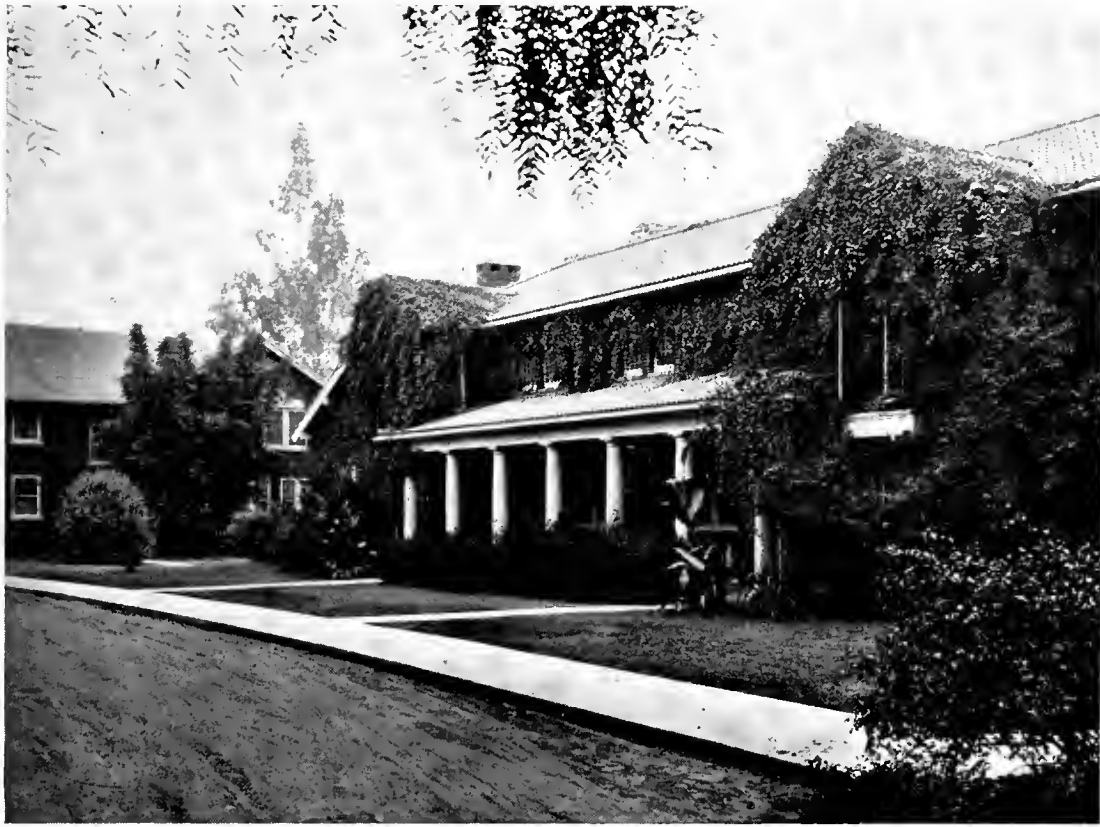
MAIN ELEVATION, HOSPITAL BUILDING
