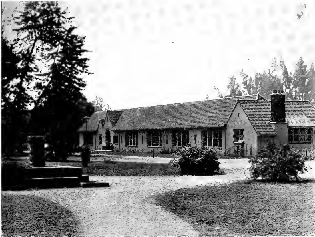
MAIN ELEVATION, SCHOOL BUILDING
