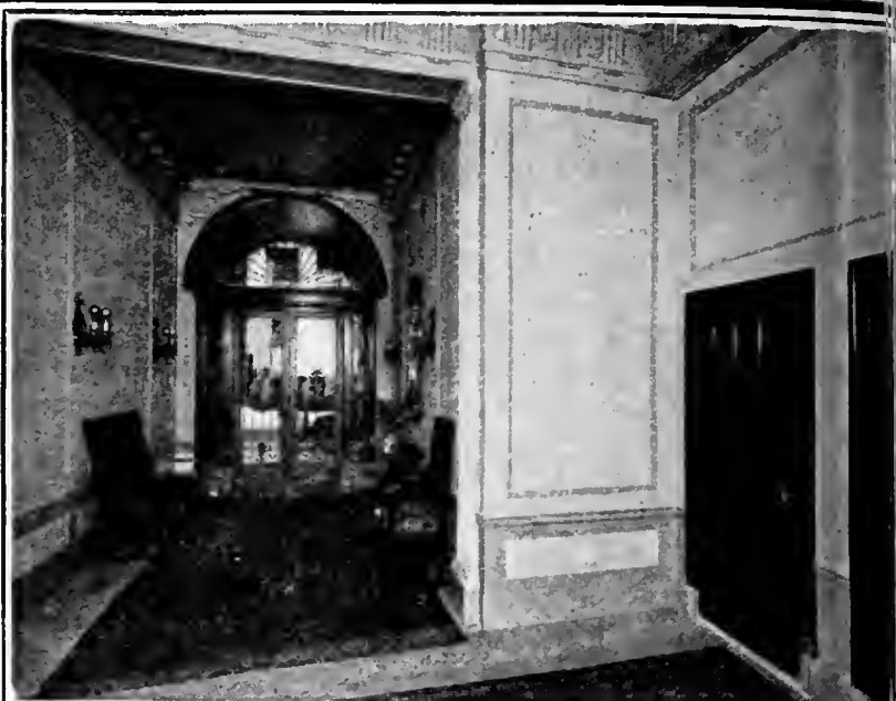
Interior View of Apartment House, 535 Geary Street, San Francisco. Walls done in Fuller Washable Wall Finish. E. E. Young, Architect, M. A. Little, Owner and Contractor.
