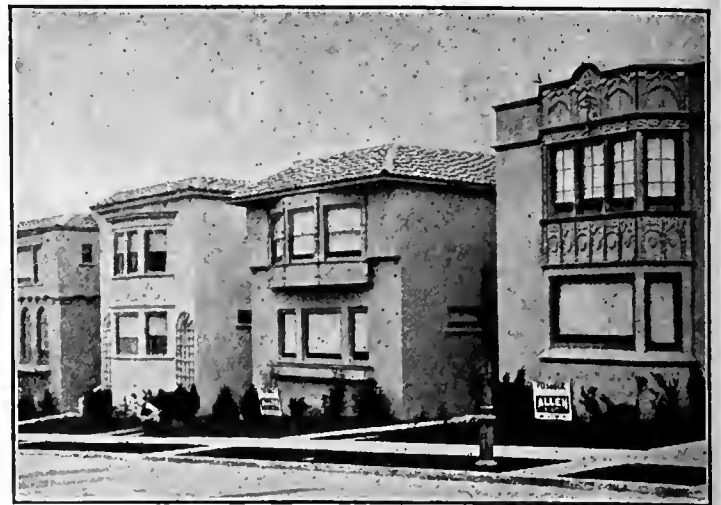
Homes at "Sea Cliff," San Francisco—exteriors finished with Concreta Allen & Co., Architects W. A. Farrell, Painting Contractor
