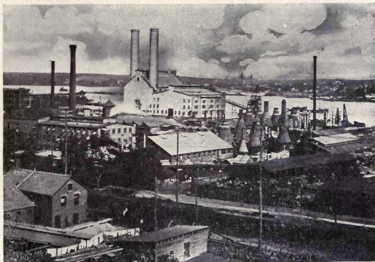
Fig. 313.—Plant No. 2 of the Atlantic Terra Cotta Company, Perth Amboy, New Jersey. By courtesy of the Atlantic Terra Cotta Company.
