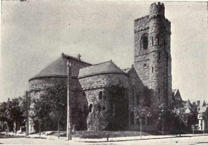
Fig. 57.—St. Paul's church, Paterson, New Jersey, built of Pompton pink granite. By courtesy of J. Volney Lewis.
