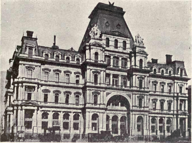
Fig. 50.—Post Office, Boston, Massachusetts, built of Rockport gray granite. Rockport, Massachusetts. By courtesy of the Rockport Granite Company.
