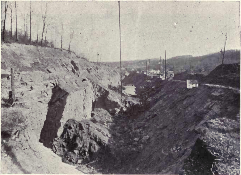
Fig. 237.—Quarry in brownstone, Hummelstown, Pennsylvania. Photo. by T. C. Hopkins.
