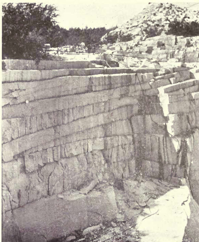
Fig. 75.—Wetmore and Morse granite quarry, Barre, Vermont, showing sheeted structure. Photo. by C. H. Richardson.
