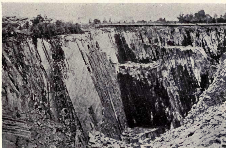
Fig. 241.—Merrill slate quarry, Brownville, Maine. The end wall working face has 42 beds of slate alternating with quartzite. By courtesy of the U. S. Geological Survey.
