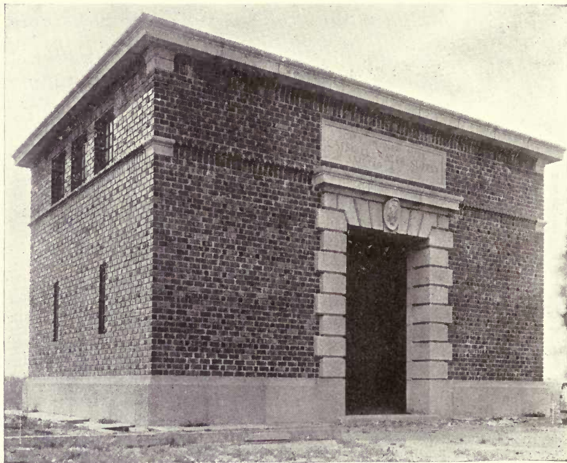
Fig. 306.—Type of building as built for the city of New York by the Board of Water Supply. H. L. Rogers, architect. Catskill aqueduct, portion of the new water system for city of New York. This brick building is trimmed with Onondaga litholite. Photo. furnished by the Onondaga Litholite Company, Syracuse, New York.
