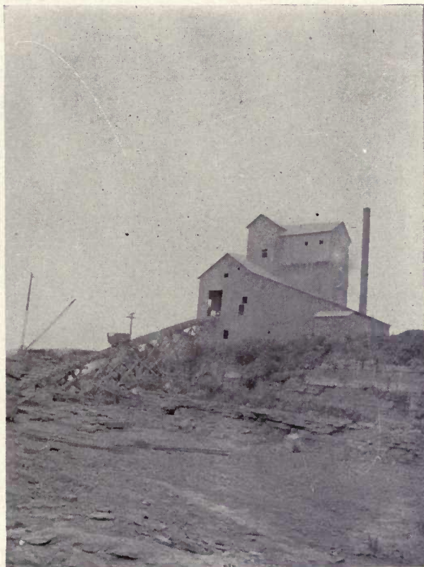
Fig. 302.—Stone crushing plant, Prospect, Oneida County, New York. Photo. by M. C. Collister.
