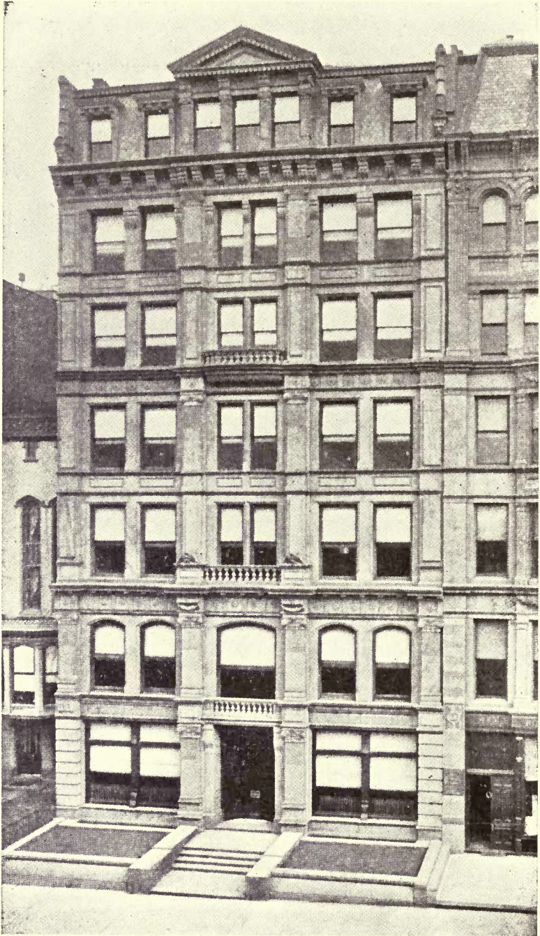
Fig. 230.—Pottier and Stymus building, New York City, showing the use of Hummelstown brownstone in brownstone fronts (entire front of dressed brownstone). Photo. by T. C. Hopkins.
