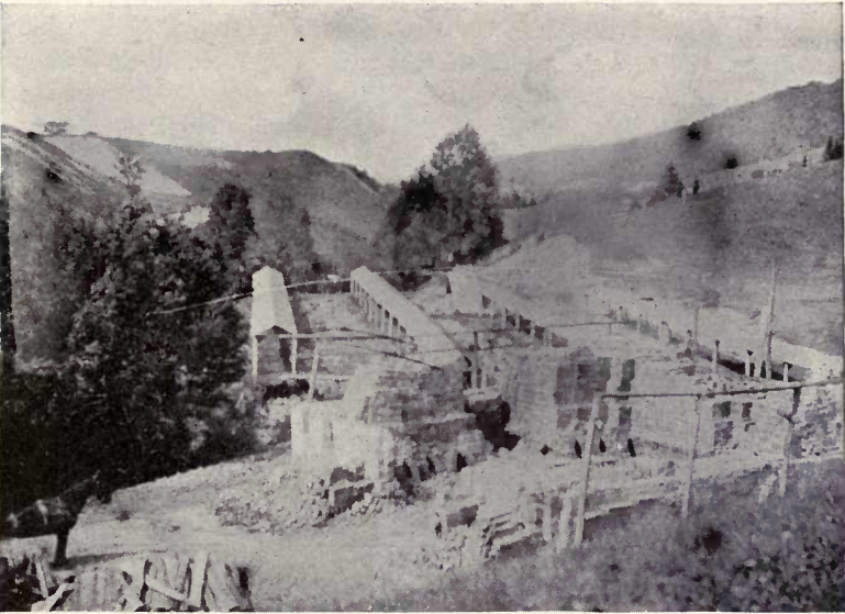
Fig. 265.—Brick yard, kiln and drying sheds, St. Johnsbury Center, Vermont. Photo. by C. H. Richardson.
