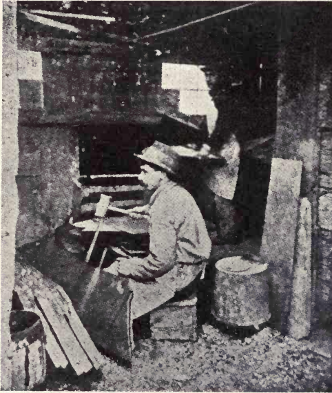
Fig. 252.—Splitting slate, Pen Argyl, Pennsylvania. Photo. by J. N. Howell.
