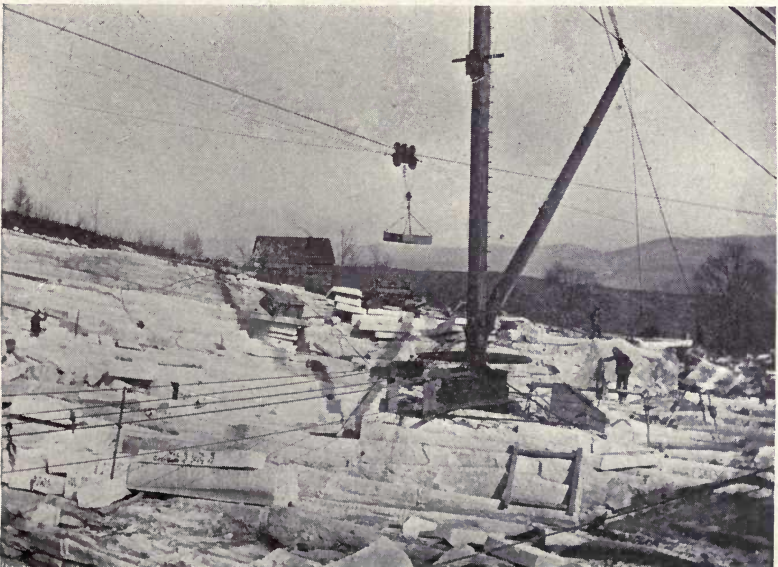
Fig. 96.—Granite quarry, Bethel, Vermont, showing sheeted structure. Photo. by C. H. Richardson.
