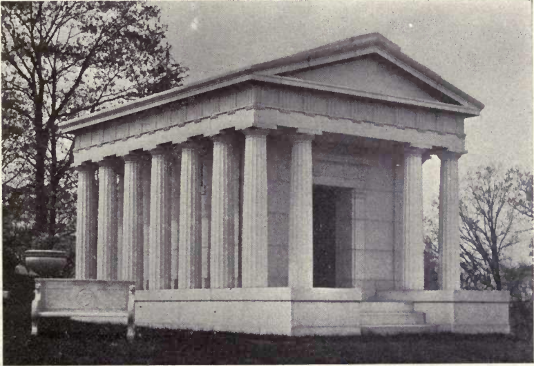
Fig. 61.—Mausoleum of Russell Sage, cut from Westerly, Rhode Island, granite and erected in Oakwood Cemetery, Troy, New York. H. O. French, architect. By courtesy of E. L. French.
