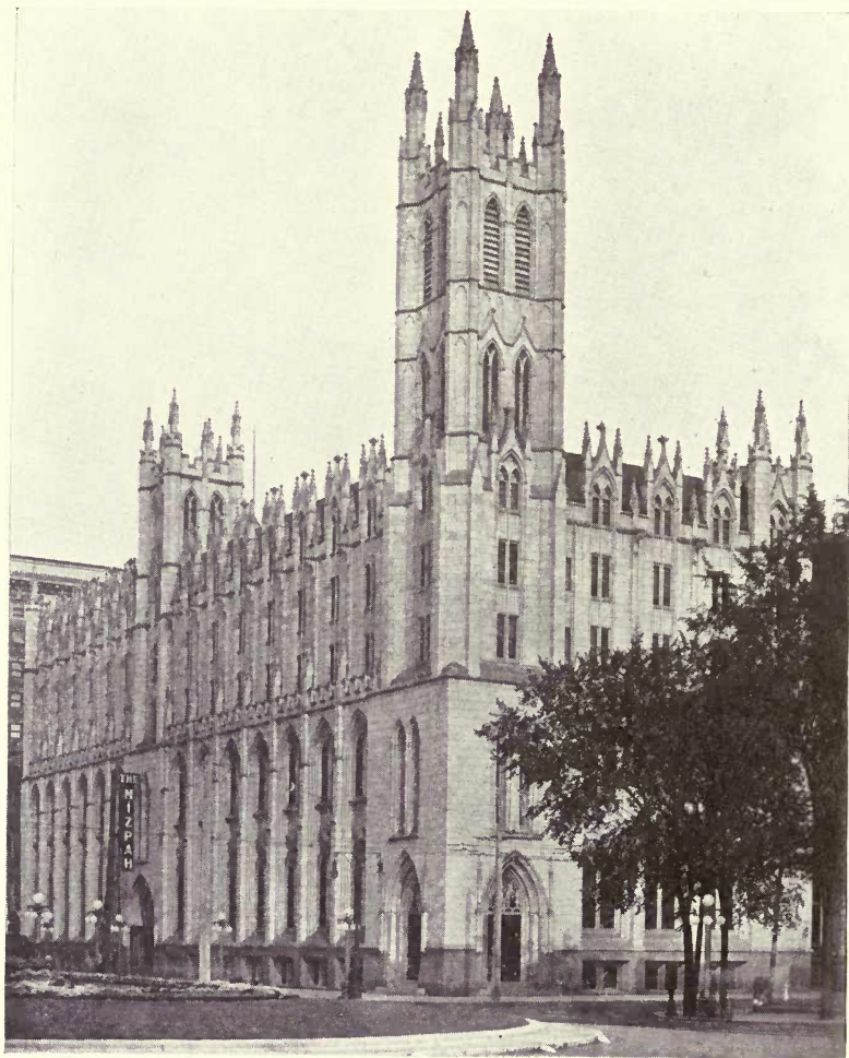
Fig. 308.—First Baptist Church, Syracuse, New York, built of terracotta. Gordon Wright, architect. Photo. by Smith and Holmes.
