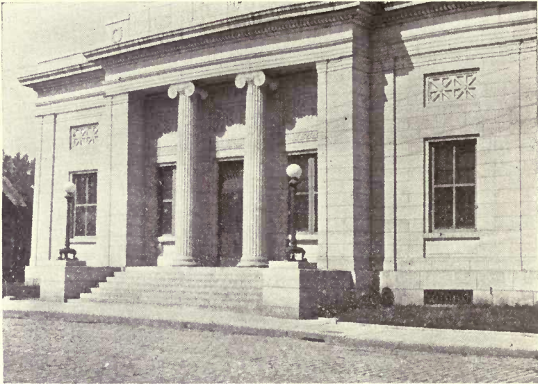
Fig. 77.—Entrance to postoffice, Barre, Vermont, built of light gray Barre granite. Photo. by C. H. Richardson.
