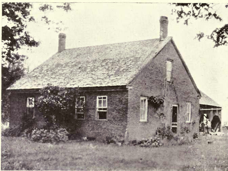
Fig. 268.—Brick house built in Calais, Vermont, in 1815, with brick manufactured from glacial clays. Photo. by C. H. Richardson.
