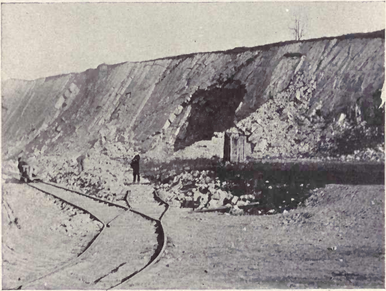
Fig. 155.—Limestone quarry at Bellefonte, Pennsylvania. Photo. by T. C. Hopkins.
