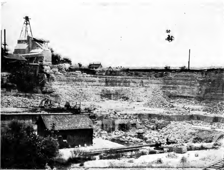
PLATE VI, FIG. 2. — General view of a limestone quarry, showing stratified character of the rock.
