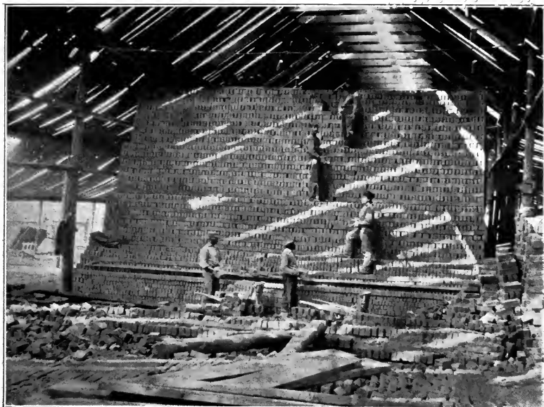
PLATE L, Fig. 1. — Setting brick for a scove kiln. (After Ries, N. J. Geol. Surv., VI, 1900.)
