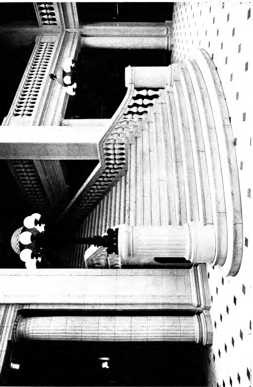
PLATE LIV. — Interior of Railway Exchange Building, Chicago, Ill. All glazed terra cotta except steps and floor which are marble. (Photo from Northwestern Terra Cotta Company.)
