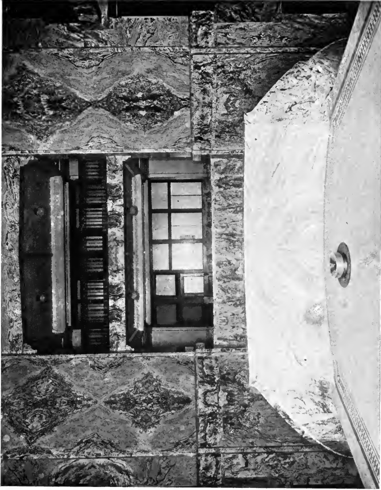
PLATE XXXV. — Interior of Harris County Court House, Houston, Tex., showing creole matched marble. (Photo from Georgia Marble Company.)
