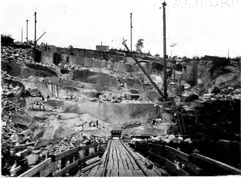
PLATE XX, Fig. 1. — Granite quarry, Hardwick, Vt.
