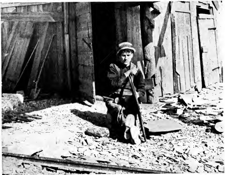
PLATE XLI, Fig. 2. — Splitting slate. (Photo by H. Ries.)
