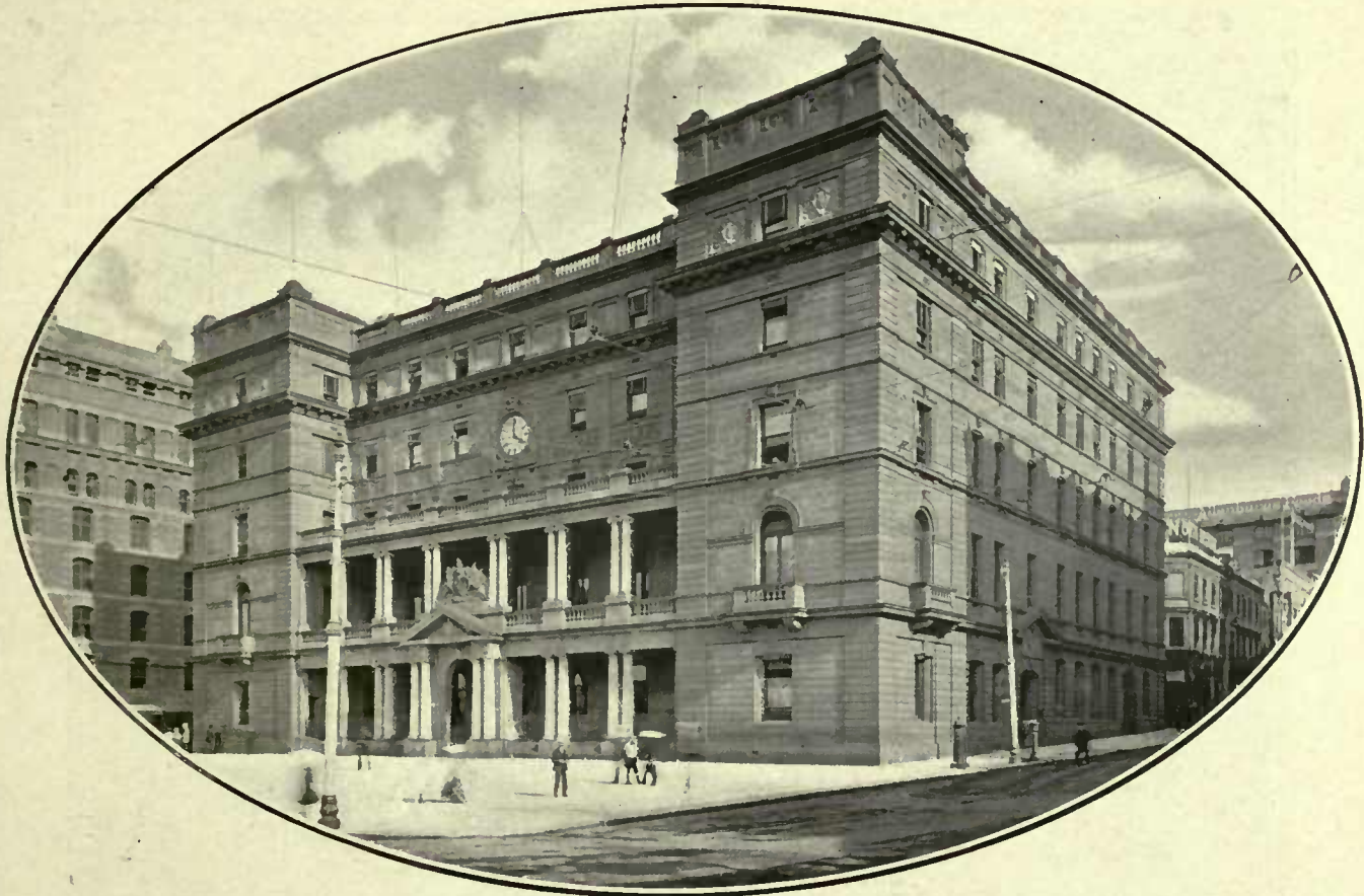
MORUYA GRANITE AND SYDNEY SANDSTONE. (THE CUSTOM HOUSE, SYDNEY, NEW SOUTH WALES.)
