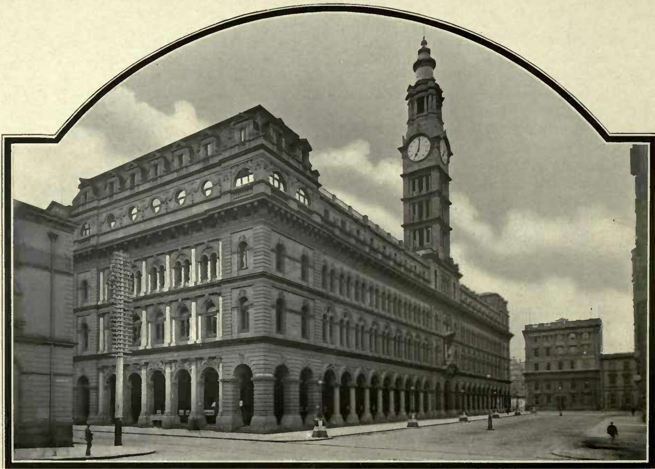
SYDNEY SANDSTONE AND MORUYA GRANITE. (GENERAL POST OFFICE, SYDNEY, NEW SOUTH WALES.)
