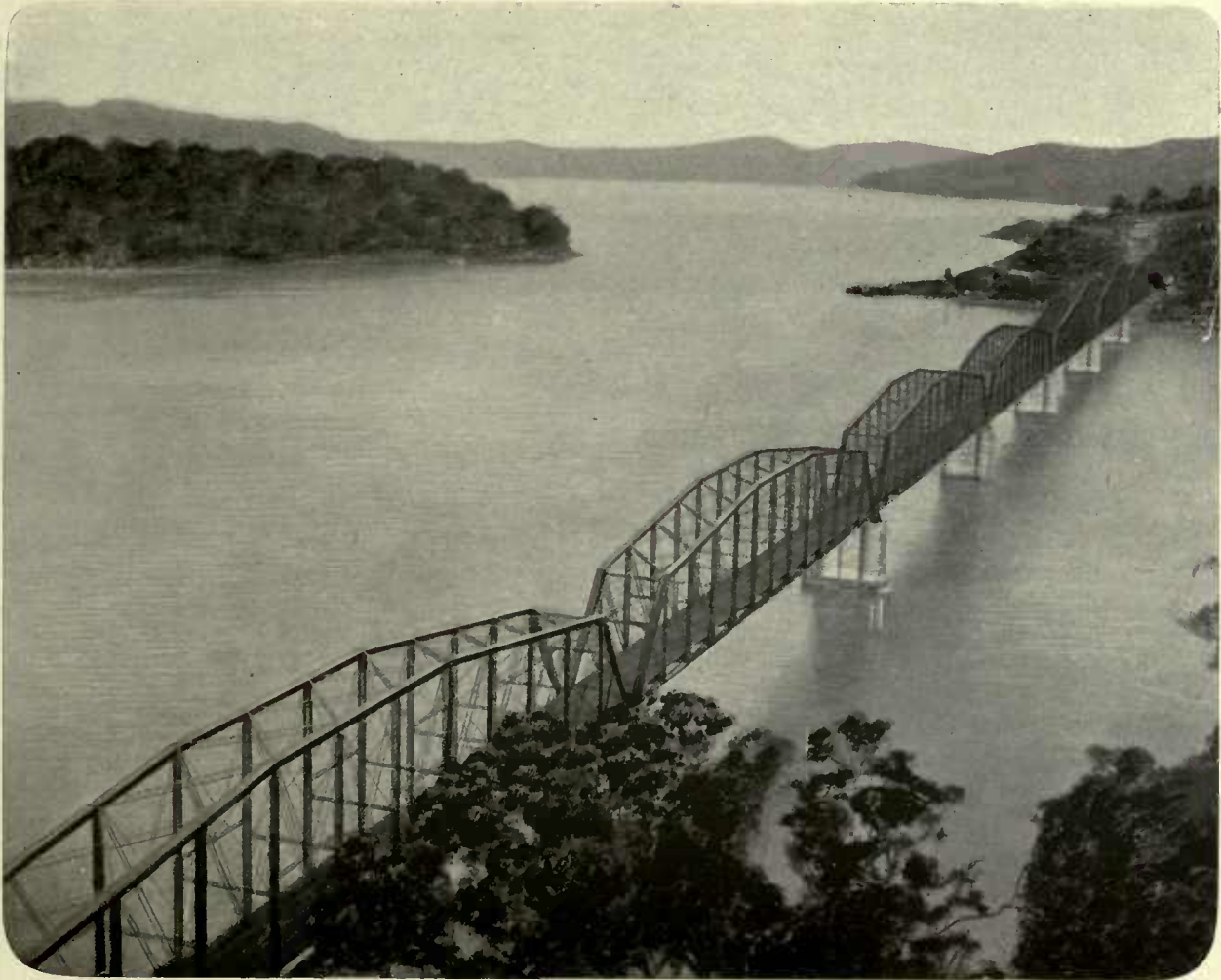
PIERS OF BOWRAL TRACHYTE. (HAWKESBURY RIVER BRIDGE, N.S.W.)
