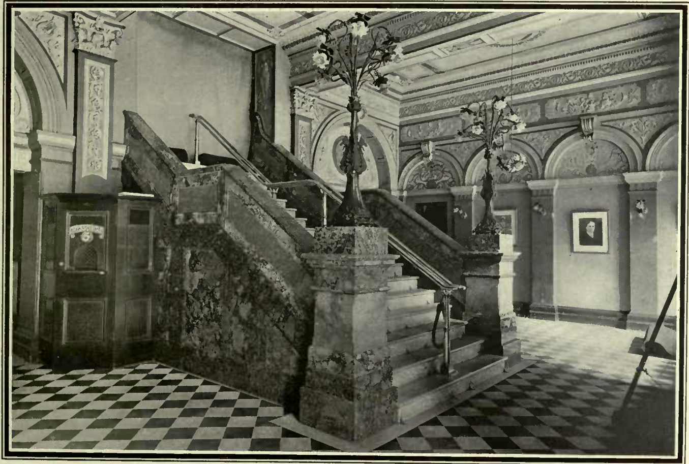
FERNBROOK MARBLE STAIRS. CALOOLA PAVEMENT. (VESTIBULE HER MAJESTY'S THEATRE, SYDNEY.)
