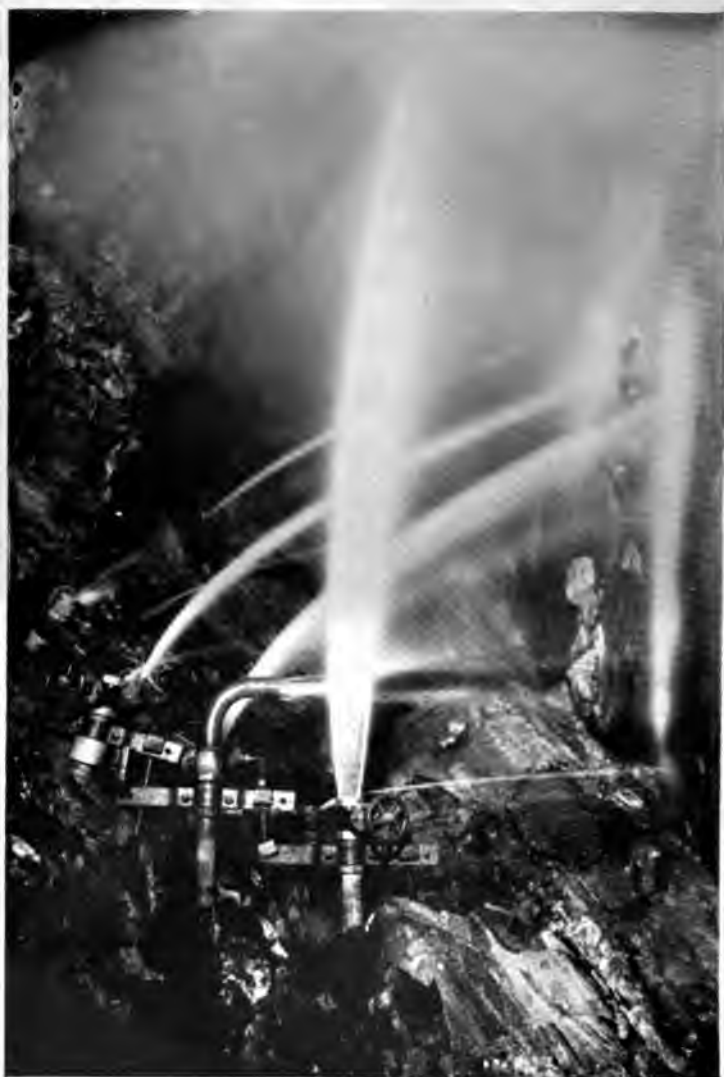
FIG. 15.—Drainage from bleeder holes, 1,150-ft. level.
