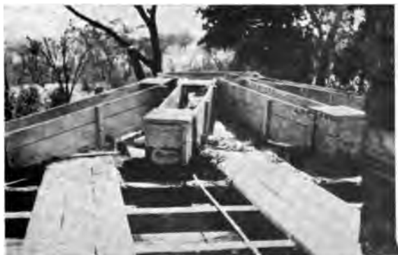
FIG. 16.—Distributor and launders feeding desliming tanks.
