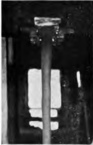
FIG. 17.—Column of sand discharging from ore gate of desliming tank.
