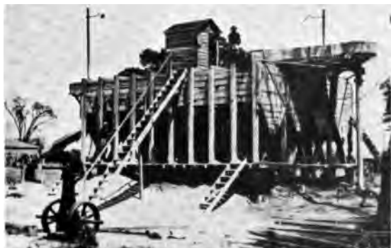
FIG. 14.—A battery of four desliming tanks.
