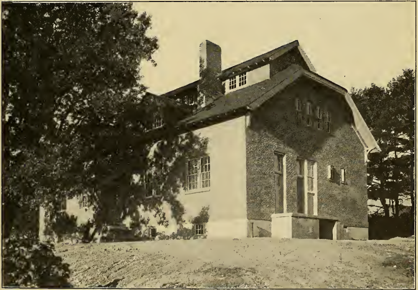
Fruit Storage Building and Laboratory, erected in 1910-11.
