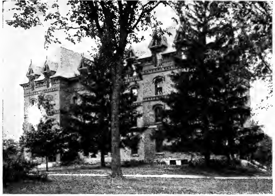
North College Dormitory
