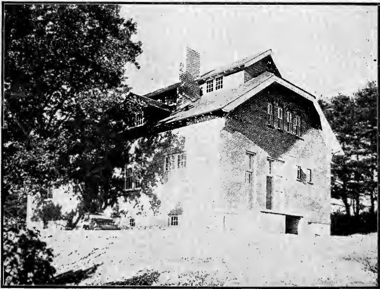
COLD STORAGE PLANT
