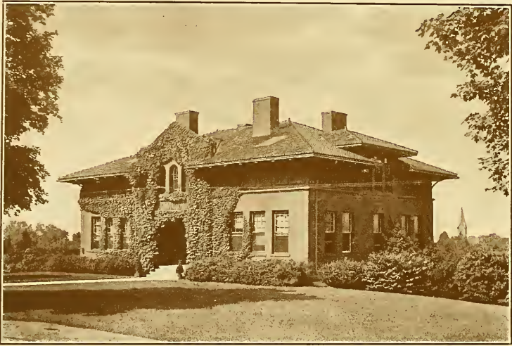
WILDER HALL is noticeable as one of the best designed and best built buildings on the campus. It is the headquarters of the Division of Horticulture, the work here being almost exclusively in Pomology and Landscape Gardening.
