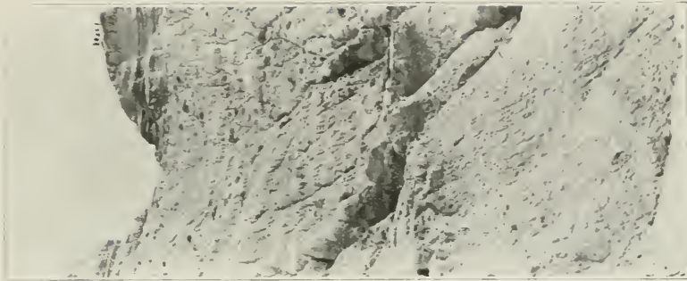
Detail of the Great Wall near Big Foot Pass.
