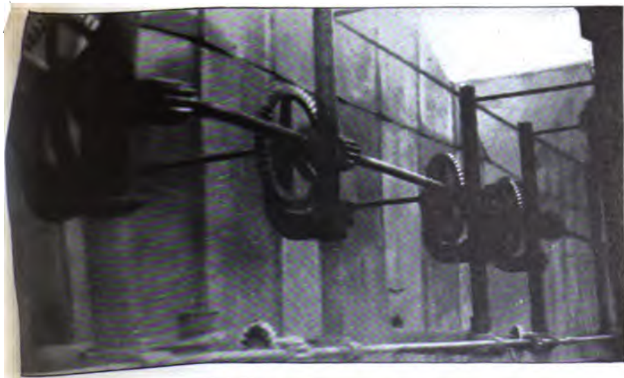
B. DRIVING MECHANISM IN ROTATING-DISK PROCESS.
