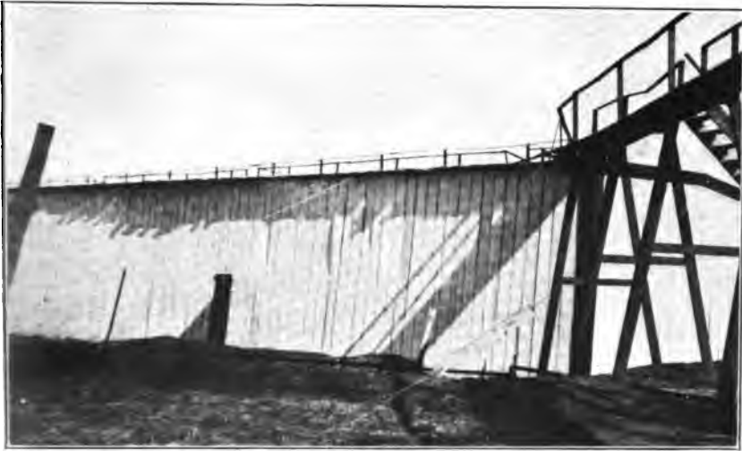
A. HOUSING FOR WOODEN LEASE TANKS.
