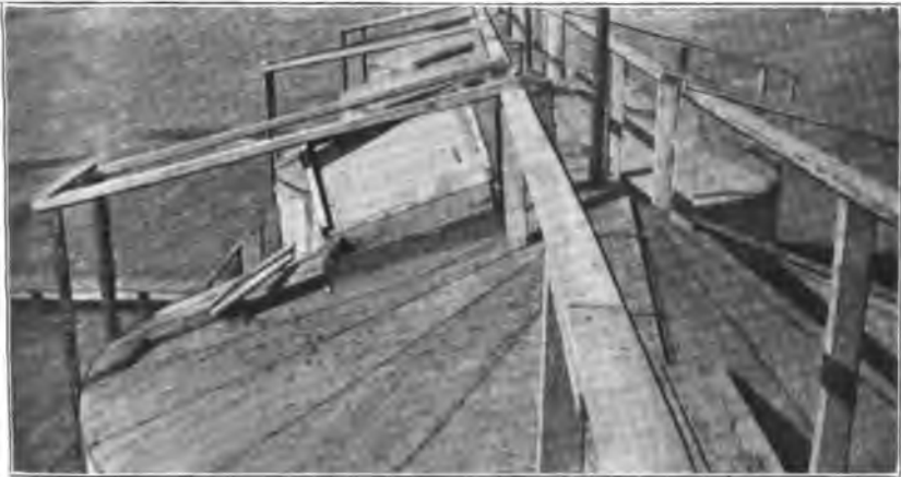
B. ROOF OF JACKETED TANK SHOWING DOOR OPEN.
