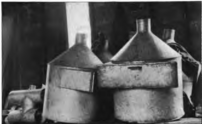
B. BOLTING MACHINES FOR REMOVING PARTICLES FROM CARBON BLACK.
