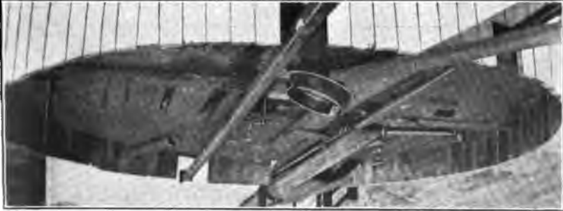
A. TOP OF JACKETED TANK BEFORE CONSTRUCTION OF ROOF.
