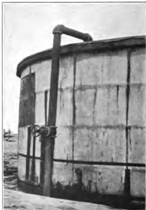
A. OVERSHOT CONNECTION FOR LARGE LEASE TANK.
