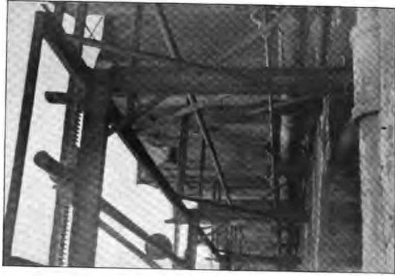
B. MAIN SHAFT AND SUPPORTS OF GAS LINE AROUND CONDENSING BUILDINGS.
