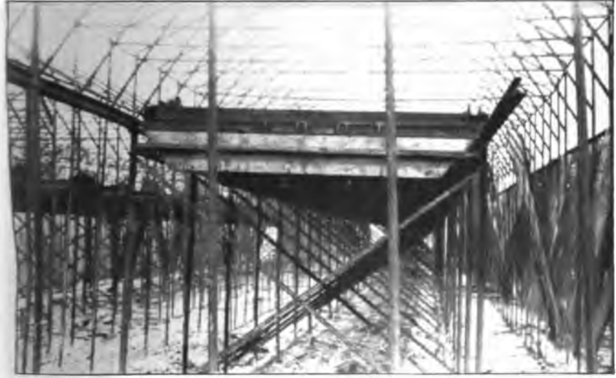
A. CHANNEL PLANT IN PROCESS OF CONSTRUCTION.
