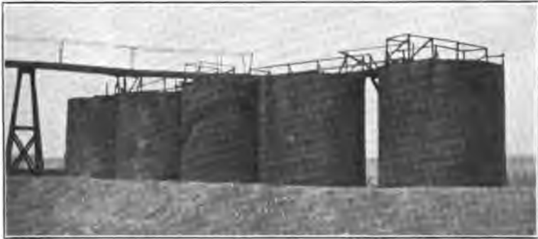
B. BATTERY OF 500-BARREL UNPROTECTED STEEL TANKS.
