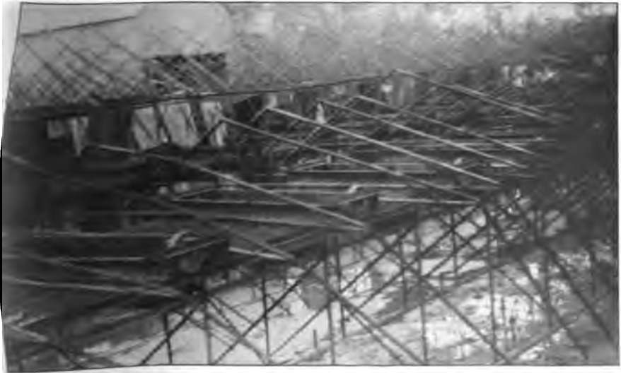
B. ANOTHER VIEW OF CHANNEL PLANT DURING CONSTRUCTION.
