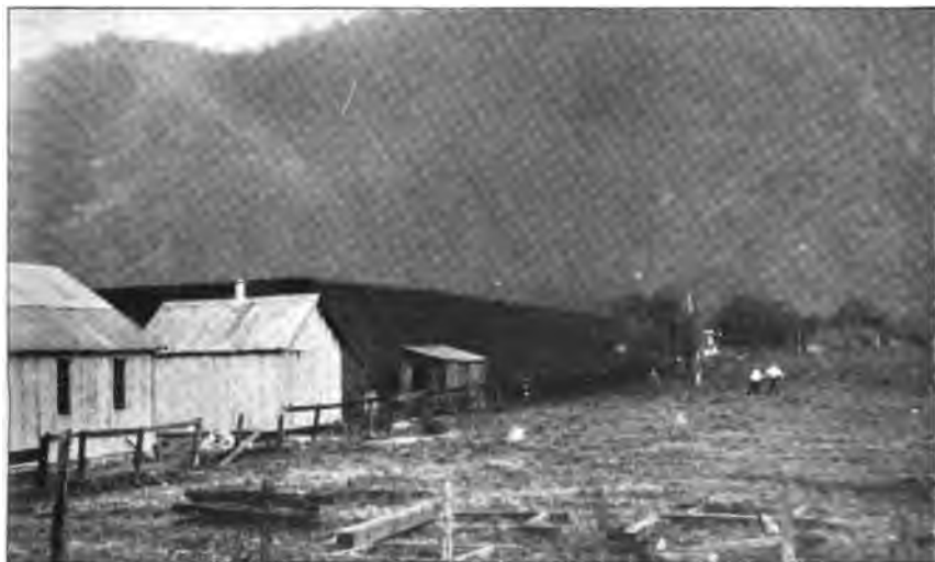
A. CARBON-BLACK PLANT EQUIPPED WITH WINDBREAK.
