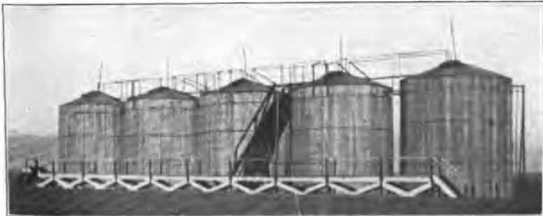
C. BATTERY OF JACKETED STEEL LEASE-TANKS.
