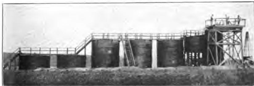
B. MEASURING-TANK SCAFFOLD ERECTED FOR DEHYDRATION TEST.
