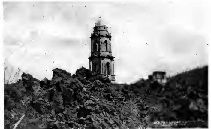
EXCEPT FOR A STEEPLE TOP, VILLAGE HAS VANISHED
