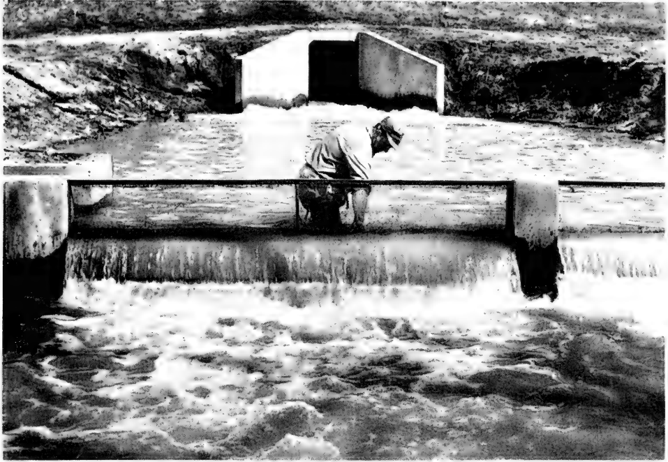
Fig. 9.—Improved type of fish screen used in draining censuses. A permanent screen was built below the outlet of Ridge Lake in 1948. It consisted of a wide concrete base, wing walls, and a center post double slotted to hold removable screen frames and planks. Planks placed below the screen frames created a head of water in the basin between the outlet and the screen and reduced the water pressure on the screen if the latter became partially clogged with debris. Screen frames could be raised for cleaning.
