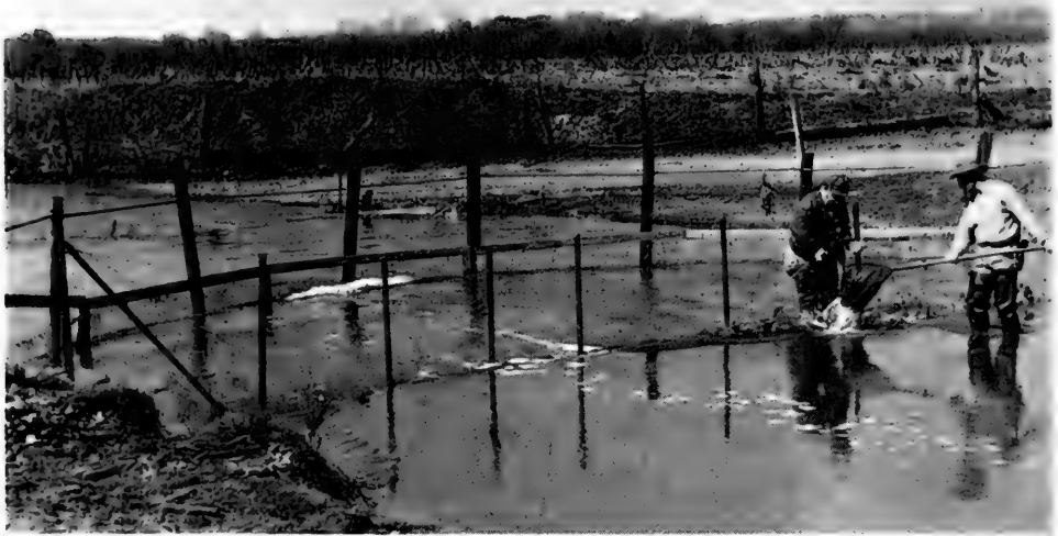
Fig. 8.—Temporary fish screen used in draining censuses. For fish censuses in 1945 and 1947, a temporary screen constructed of 1-inch-mesh poultry netting was installed across the stream channel below the outlet of Ridge Lake.
