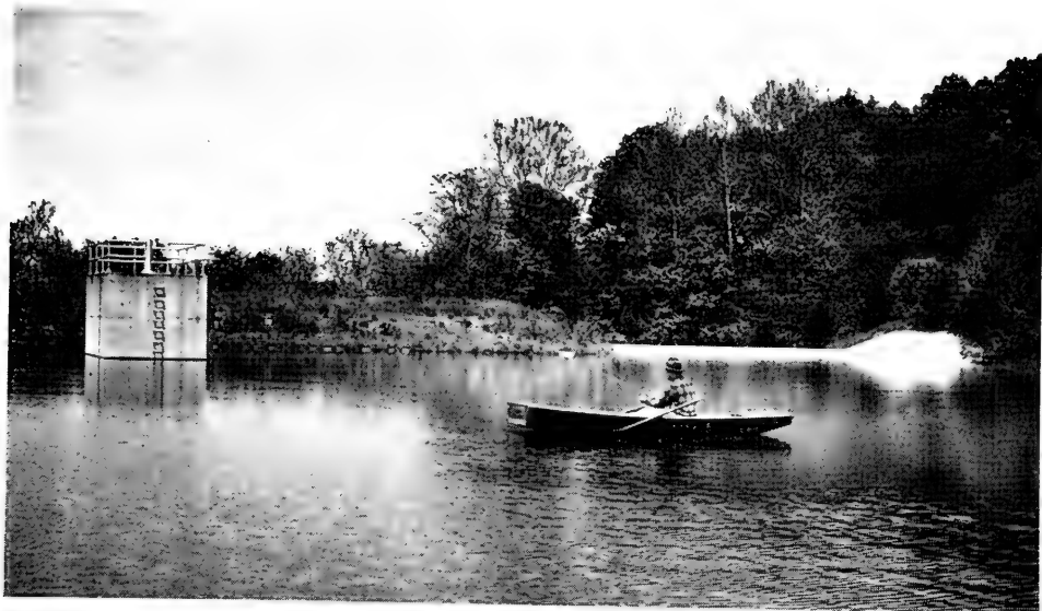
Fig. 2.—The dam, tower spillway (left), and surface spillway (right) as seen from the surface of Ridge Lake.
