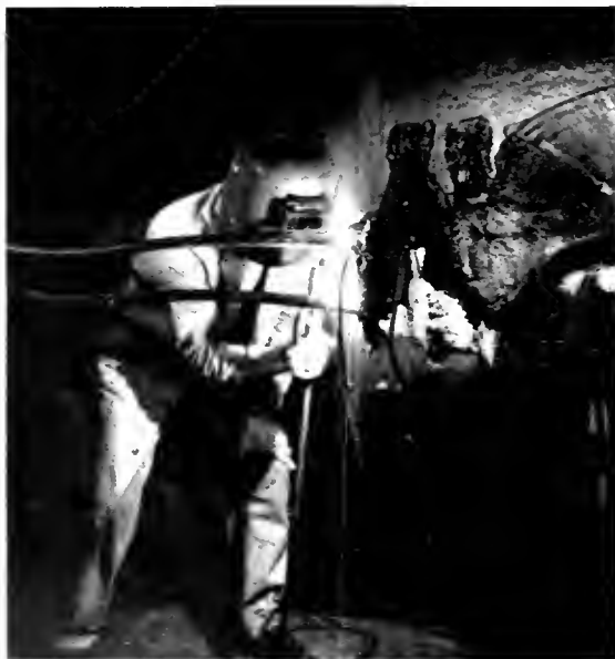
6. Metal discs that separate vertebrae are welded into place.
