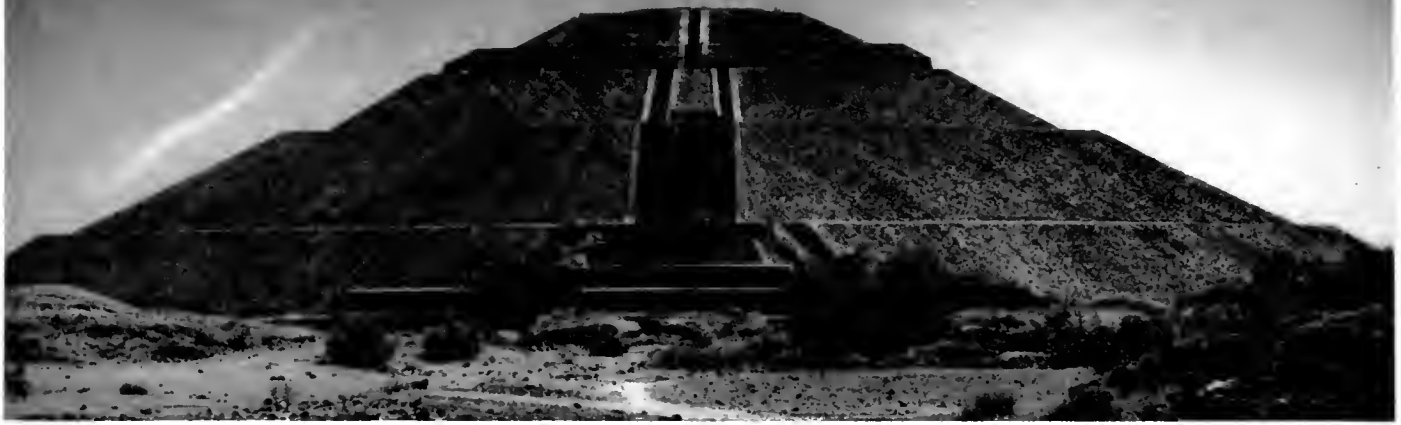
Pyramid of the Sun at TEOTIHUACAN. A view of the central stairway is shown on the cover. This stone-faced structure 200 feet high and 700 feet on a side was the base for a temple, now disappeared. The ancient city flourished from A.D. 100 to 700 and at its height contained 50,000 to 100,000 inhabitants.
