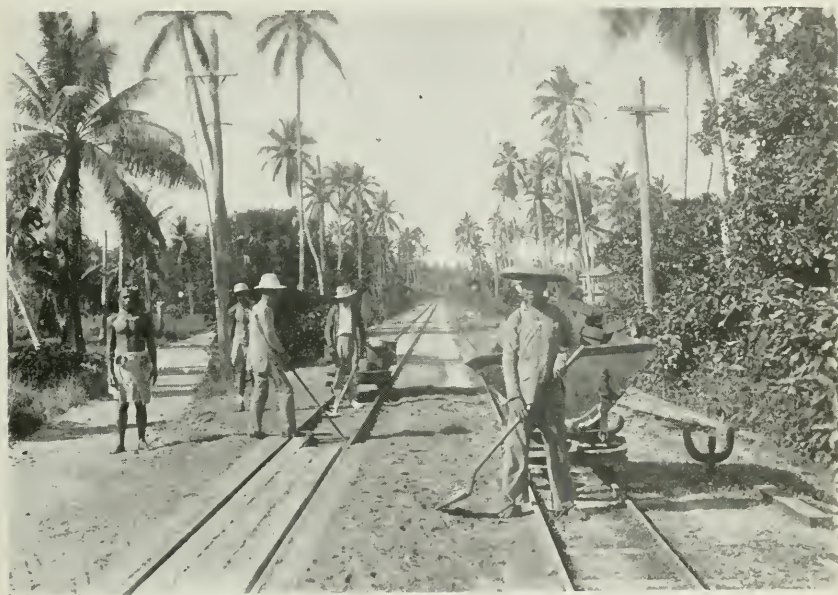
ALONG THE RAILWAY LINE.
