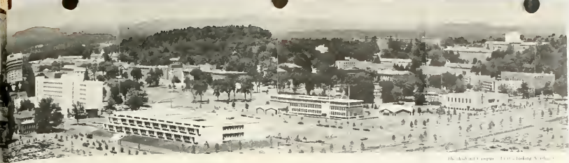
The Lowell Campus - Looking North
