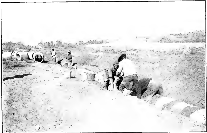
Fig. 19.—Laying 20-inch cement pipe in shallow ditch at Continental.
