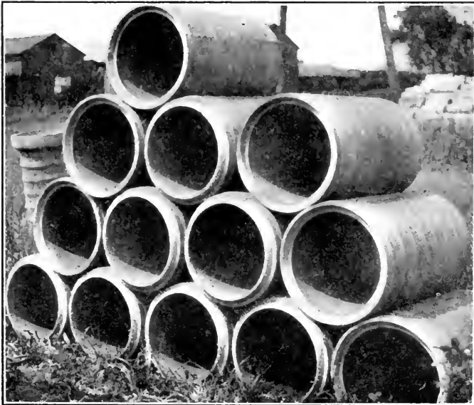
Irrigation pipe with tongue and groove joint.
