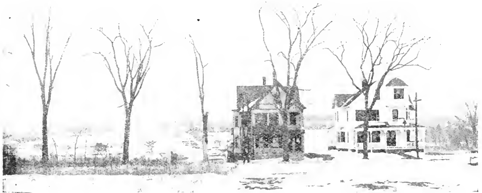
Fig. 19. Large elms killed by escaping illuminating gas, one and one-half years after leakage occurred. From "Park and Cemetery."
