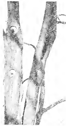
Fig. 11. Showing tree properly bolted, washer countersunk and imbedded in cement. From "Park and Cemetery."
