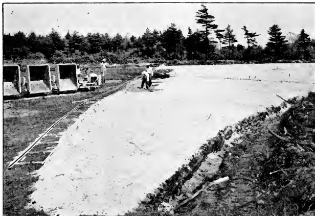
Fig. 13. Sanding a New Bog with Gasoline Engine and Cars.
