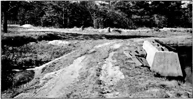
Fig. 10. A Covered or Trunk Gate.
