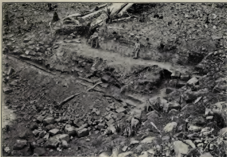
A. BEGINNING OF EXCAVATION IN TEMPLE COURT
