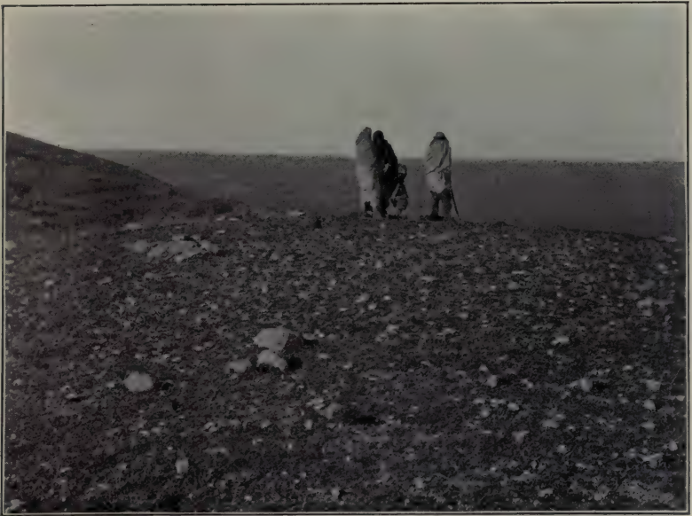
APSE BUILDING BEFORE EXCAVATION, LOOKING NORTHWEST (December 28, 1910)
