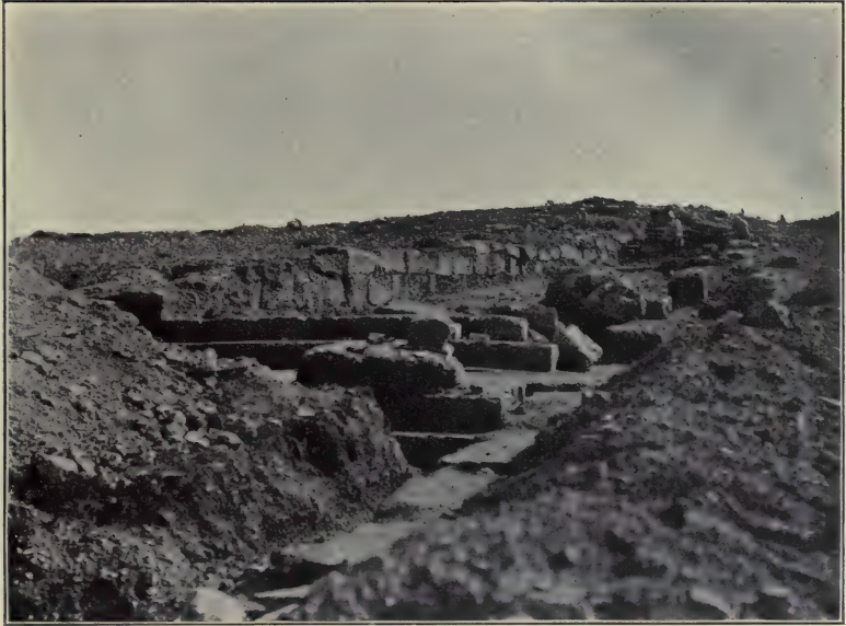
ROADWAY ON WEST SIDE OF EXCAVATION
