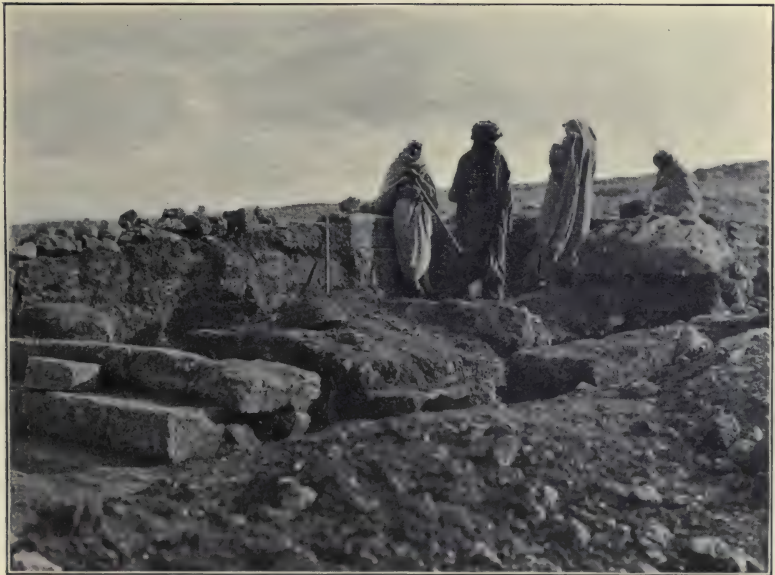
NORTHERN END OF ROADWAY (P. 153)
