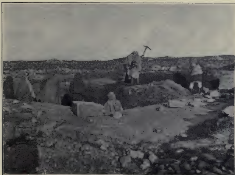
FOUNDATIONS SOUTH OF COLONNADE BUILDINGS (December 22, 1910)
