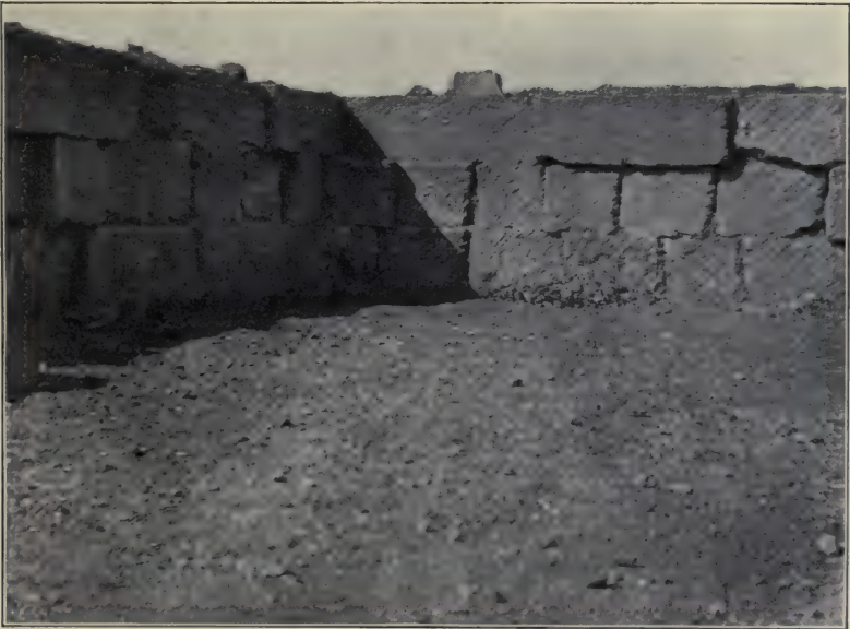
FOUNDATIONS SOUTH OF COLONNADE BUILDINGS (February 23, 1911; p. 154)
