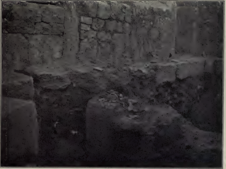
WALL OF CORRIDOR, SHOWING CONSTRUCTION (View taken at foot of west stairs)
