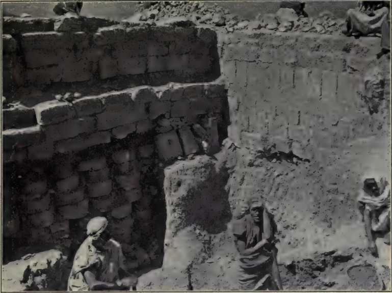
APSE BUILDING: NORTHWEST CORNER OF CENTRAL ROOM (March 27, 1911)
