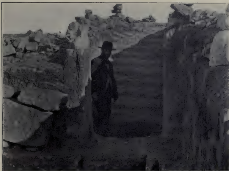
STAIRWAY IN WEST WING (P. 153)
