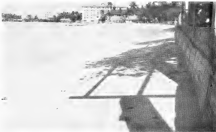
FIGURE 8. BEACH BEHIND OFFSHORE BREAKWATER, 1947
