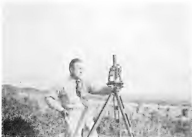
FIGURE 3.-METHOD OF OBSERVING WAVE DIRECTION
