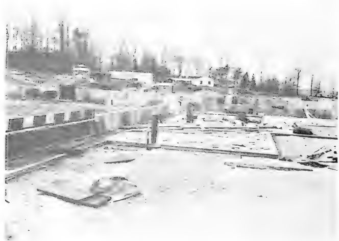
FIGURE 5. COAST MODEL TEST BASIN PERIMETER WALL AND FLOOR SLAB.
